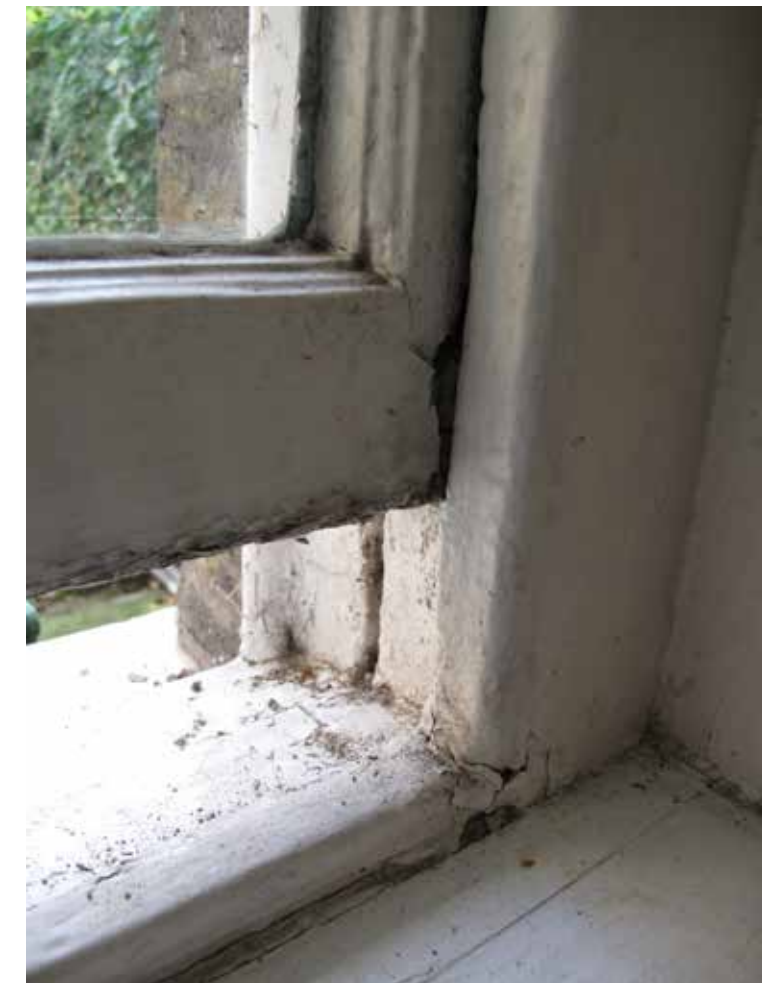
Corner of window showing poor condition
