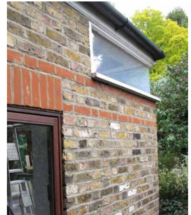
High level flimsy plastic window
