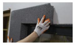
14. When working to an external corner overlap EPS boards and extend past corner (cut off flush when cured).
