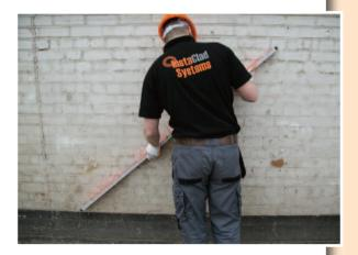
2. Starter Tracks - For standard DPC mark out a straight line using level, laser or string line. Work as close to the DPC without penetrating it (always work above DPC level). For non standard DPC please refer to site specific method statement or contact your technical inspector. Using marked out guide line and starter track as reference, drill pilot holes into substrate.
