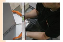
9. Fill the gap between the starter track and substrate with PU Filler foam.
