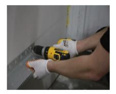
Use packing shims to adjust depth of starter track giving you a clear working line up the substrate. Ensure you have enough room for turbo fix considering the maximum working depth is 20mm.
