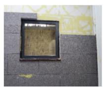
13. When installing around doors & windows an "L" shaped EPS board must be installed to avoid joints at stress points.
