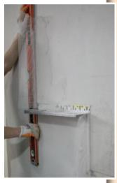
Above bay windows, porches, and garages – for example the starter track typically fitted as above but always refer to your site specific method statement. Remember to add or adjust lead flashing (where applicable) to ensure rain water runs away from rendered walls.
