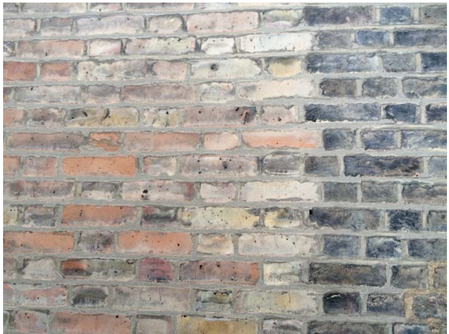
Existing light and dark brickwork interface
