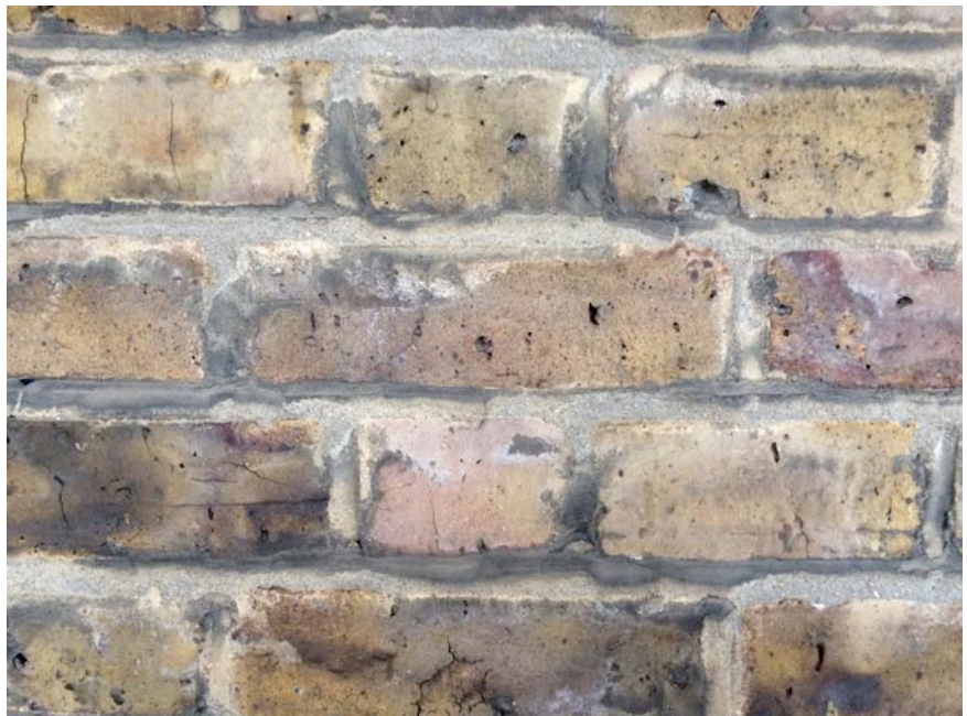
Existing brickwork to be coloured
