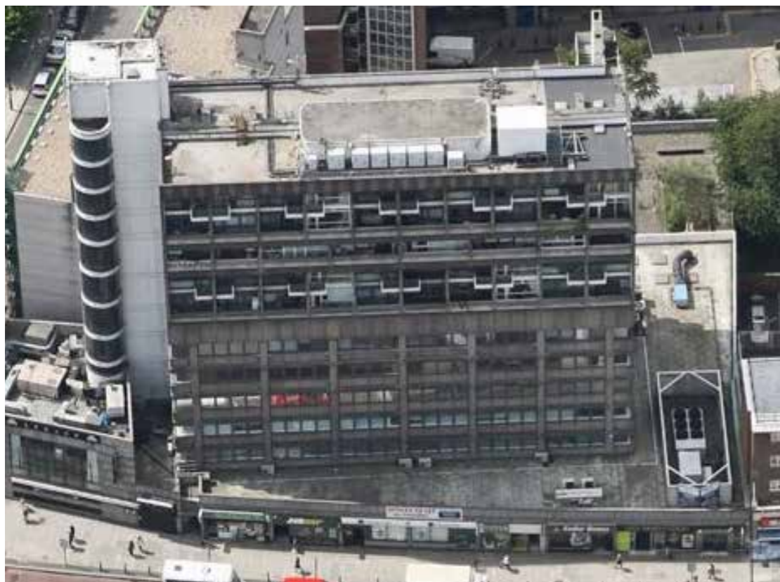
Aerial view of Centre Heights showing existing rooftop plant
