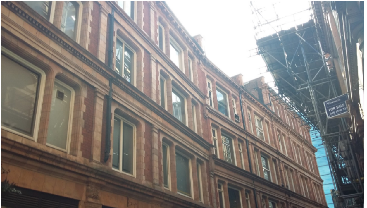
3. View of roof line
