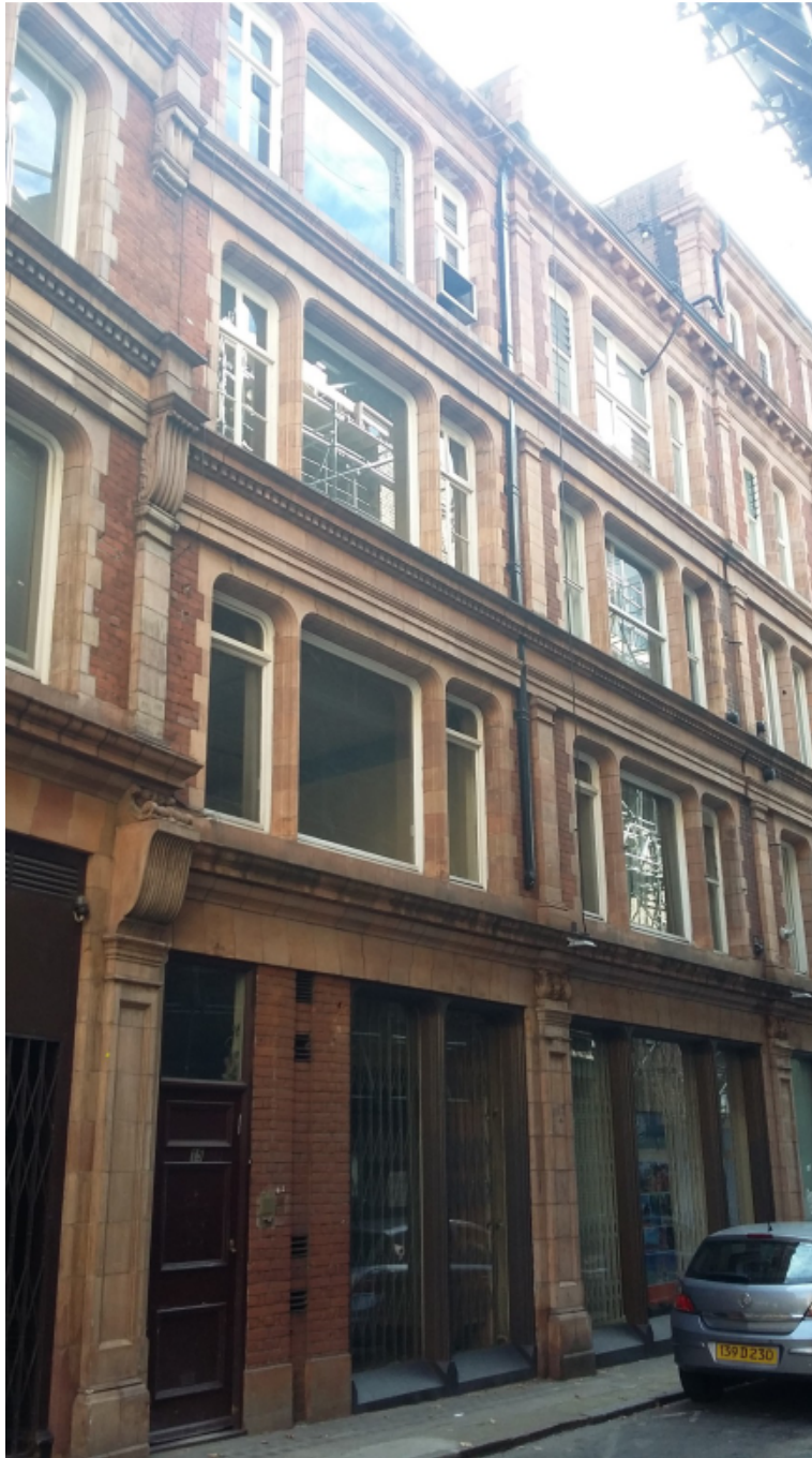
1. View of front of building
