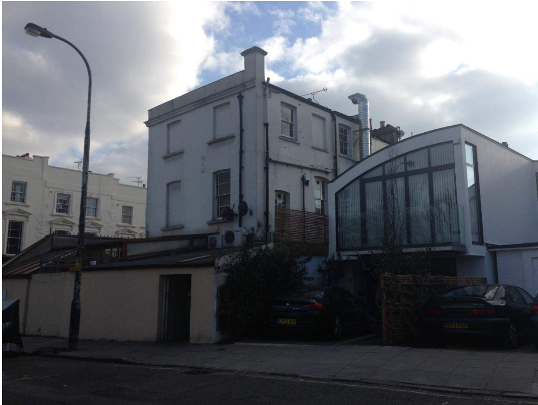
Plate 3: The two storey private residence (right) to the north of the Little Bay site (left) Looking South-West
