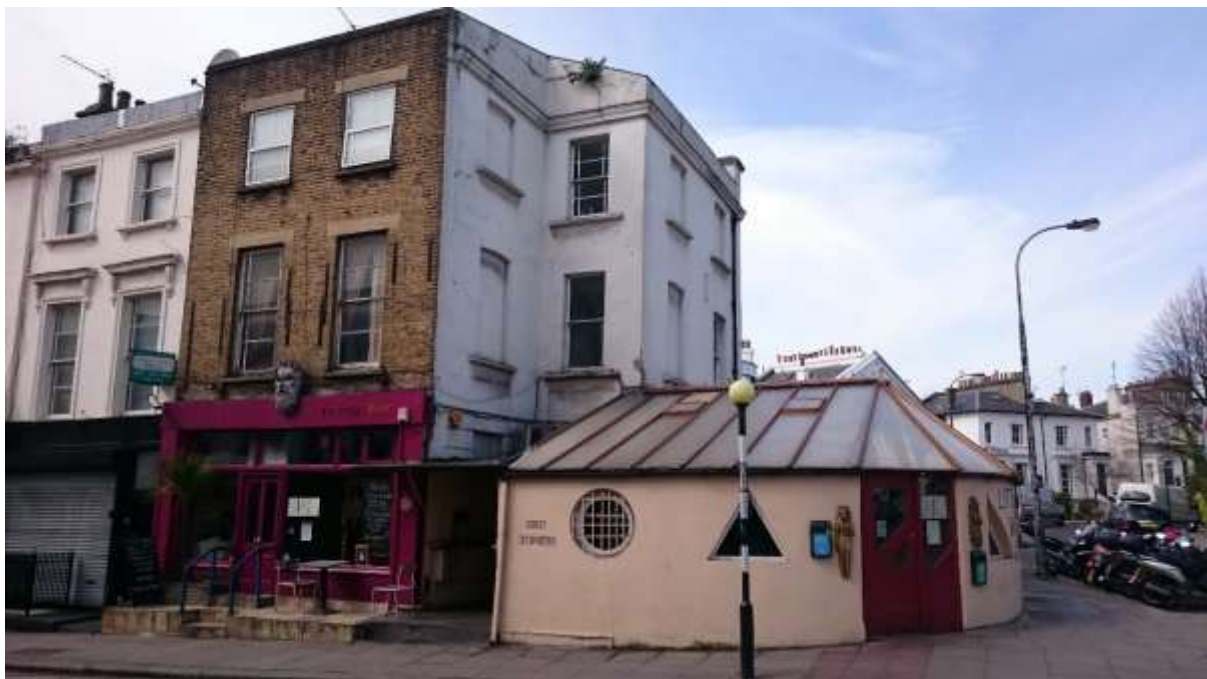
IMAGE 1: The Subject Property, illustrating the existing single storey side extension (Author's Photo)
