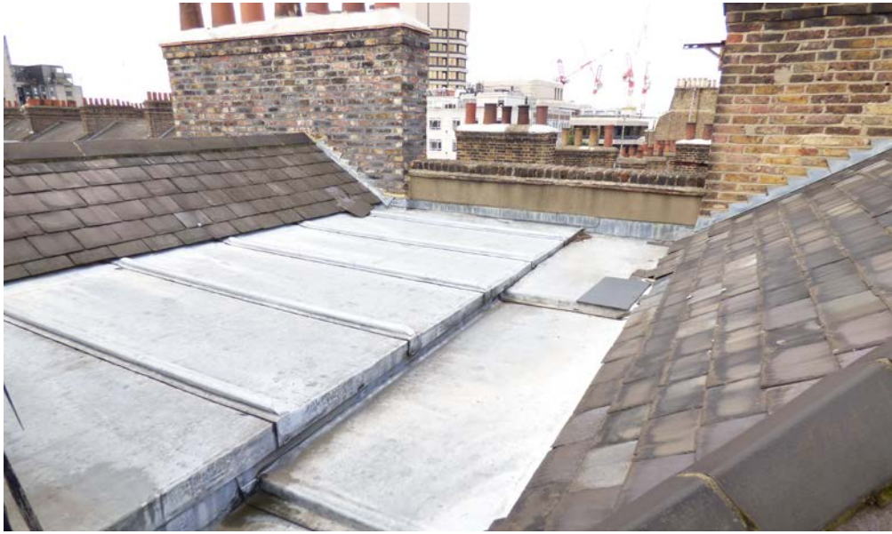
Roof Area – A/C units
