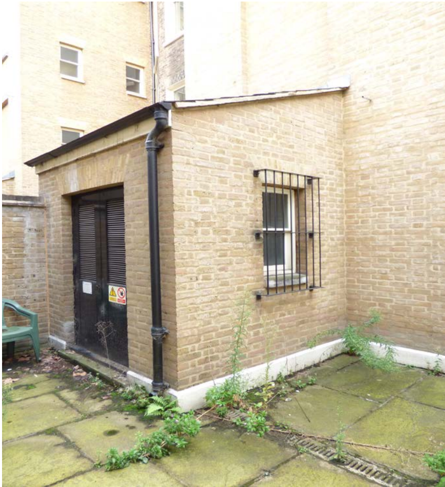
Rear area – Extension
