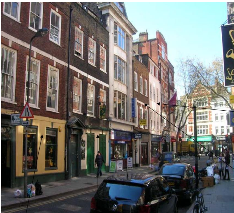
Photograph 6: Denmark Street (South Side)
