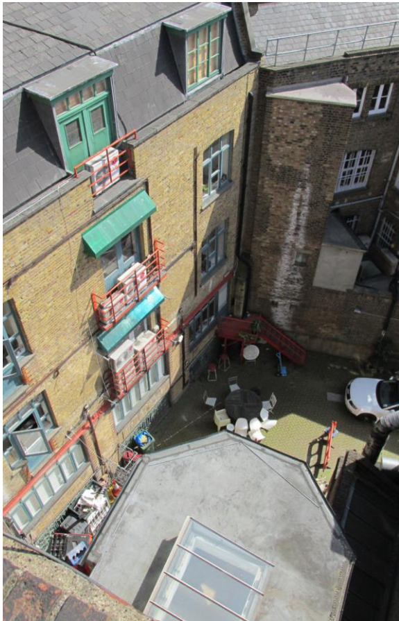
Photo 9: View of 1 Brook Mews Courtyard
