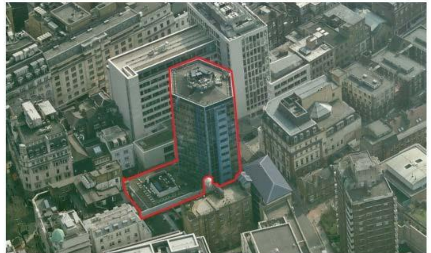
Aerial View towards the south
