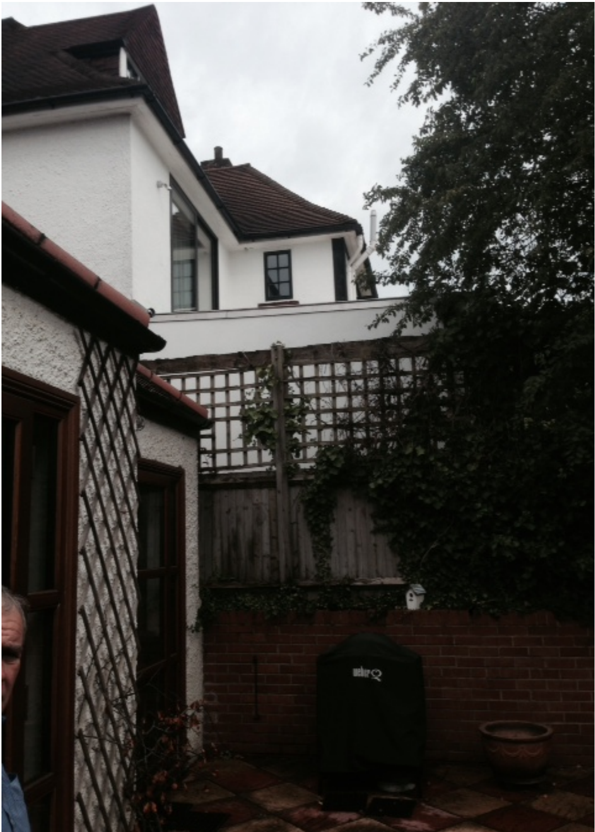
Photo F – Kitchen and garden area after the extension
