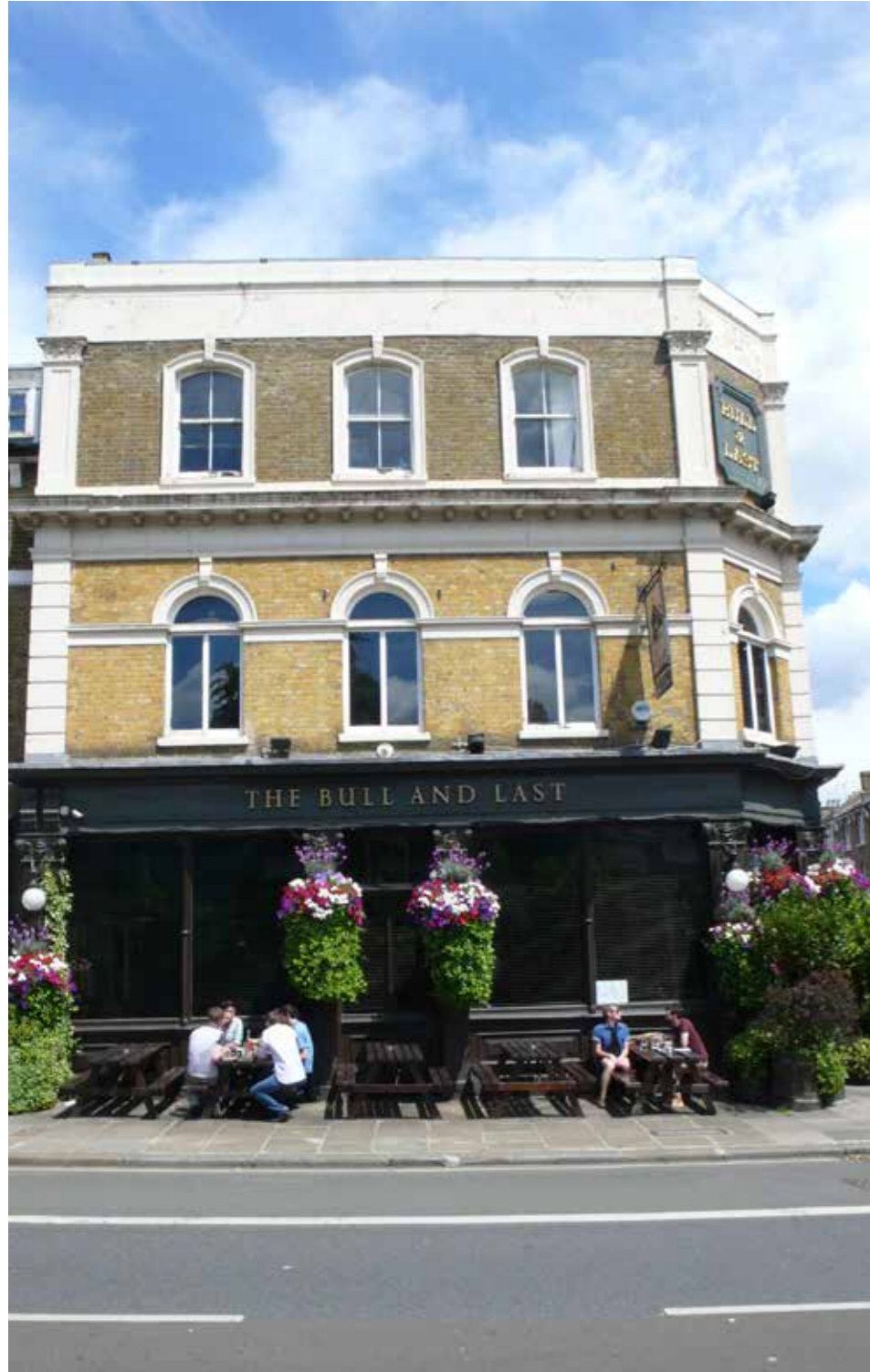
View of the building from Highgate Road
