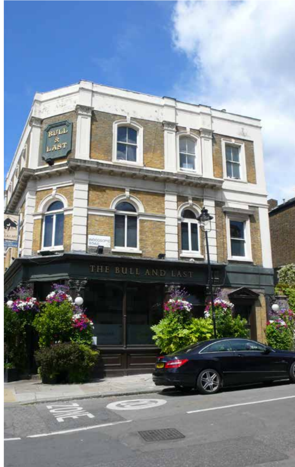
View of the building from Woodsome Road
