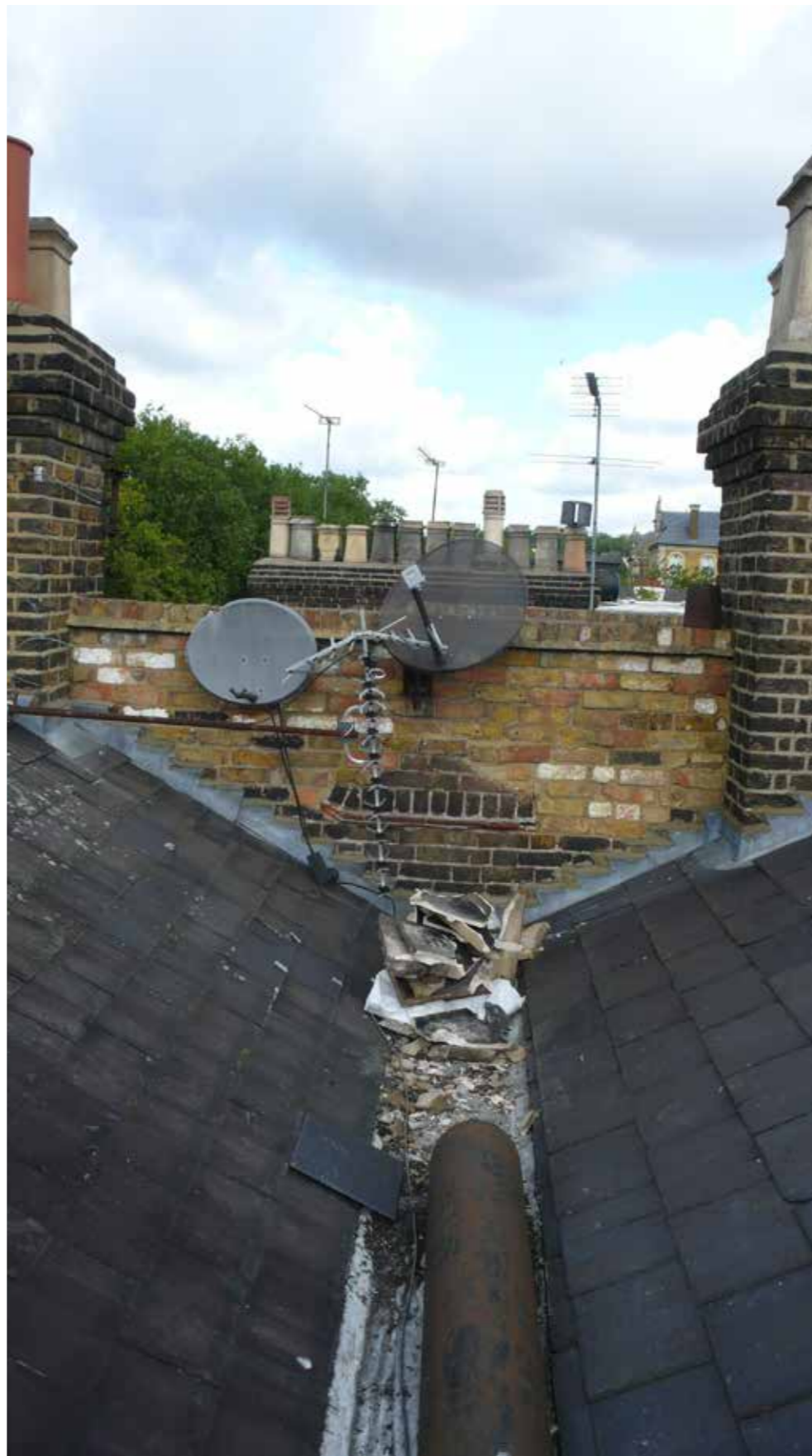
View of the existing valley roof
