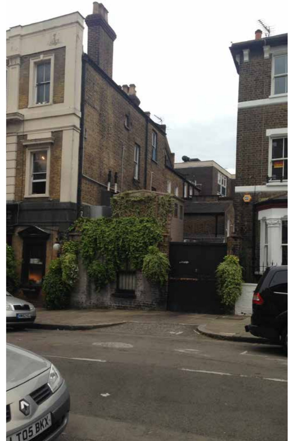
View of the building from Woodsome Road
