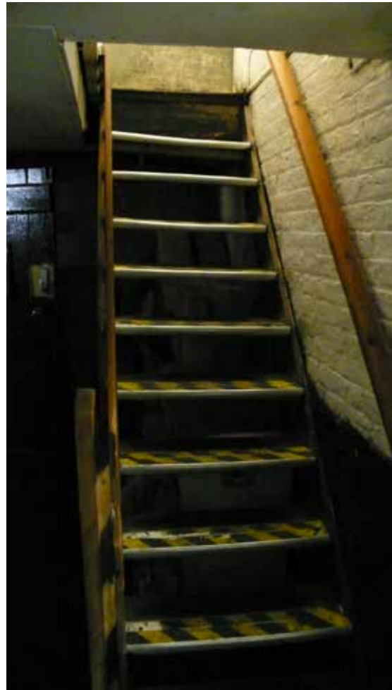
Existing basement stair
