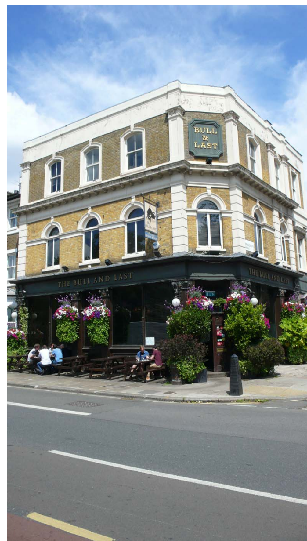
03 VIEW FROM HIGHGATE ROAD
