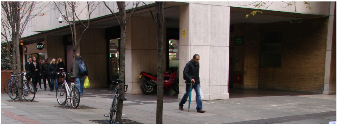
view 2 : existing A1 shop frontage and undercroft
