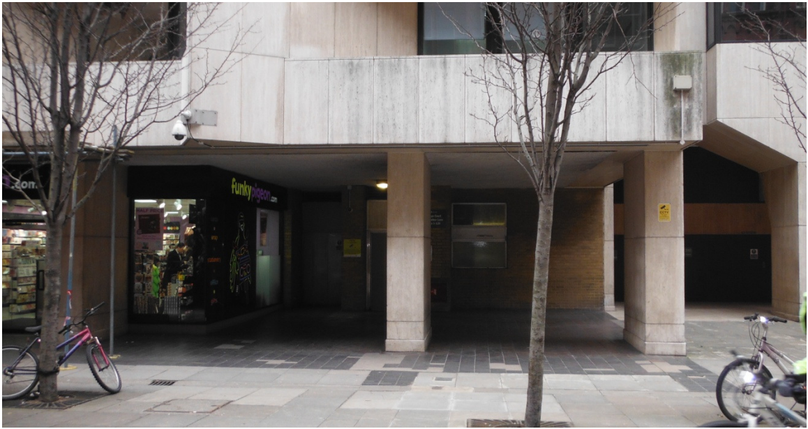
view 1 : existing A1 shop frontage and residential entrance
