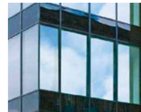
PILKINGTON Spandrel Reflective Insulated glass panels to Conway Street elevation, also to the lightwell.
