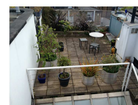
Existing Railings on terrace
