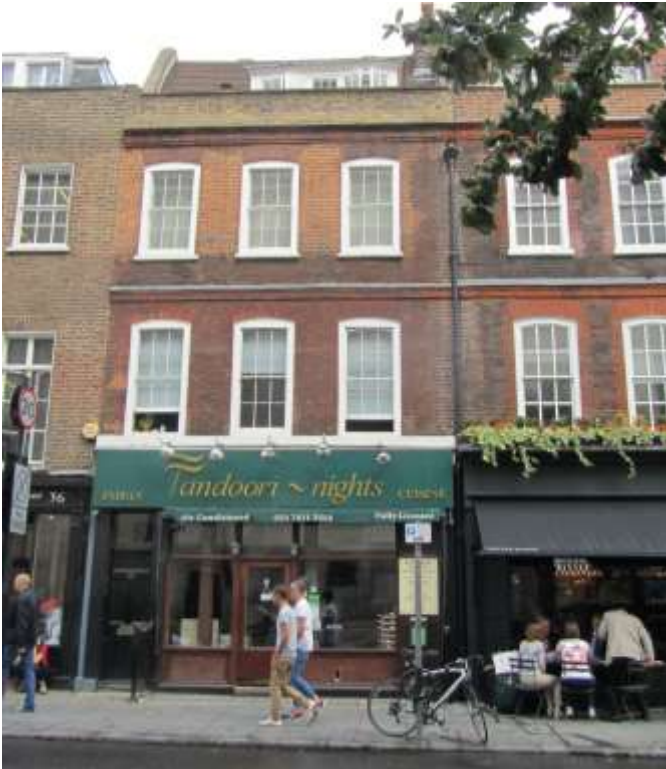
Existing signage with 5 lights above
