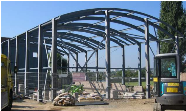
Pile Foundation, Hampton Hill
