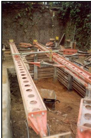
King post construction and temporary propping
