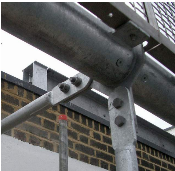
Galvanised Steel Hanger Connection Wimbledon Bridge, Wimbledon
