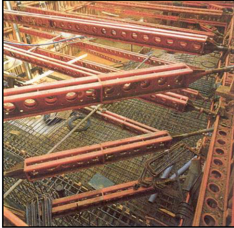
Propping to temporary retaining wall.
