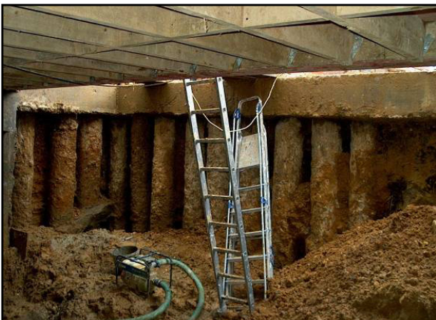
Contiguous bored pile retaining wall and capping beam.
