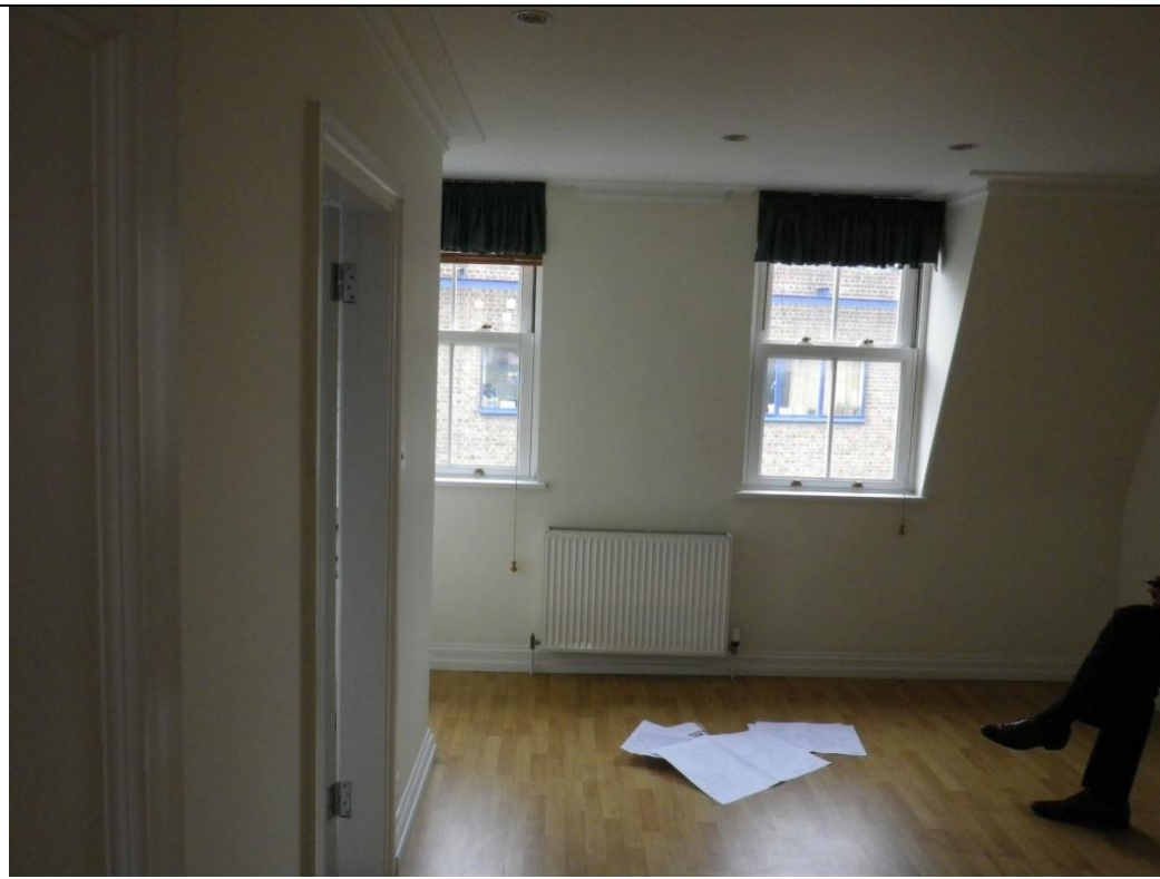
View – Inside Flat 4 in mansard of 69 – 71 Farringdon Road
