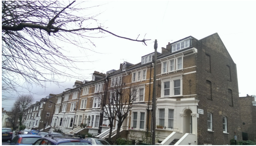
Above: a series of similar front dormer enlargements along Montpellier Grove (#43 shown on the right)
