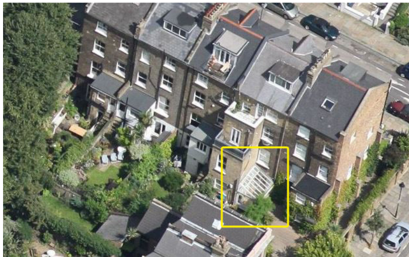
Above: an infill extension shown at the rear of 45 Montpelier Grove
