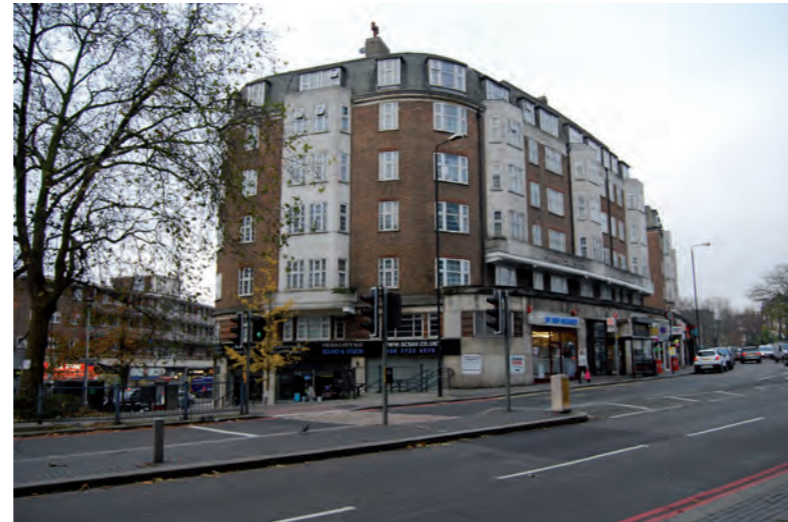
E3. Photograph of existing corner facing Swiss Cottage
