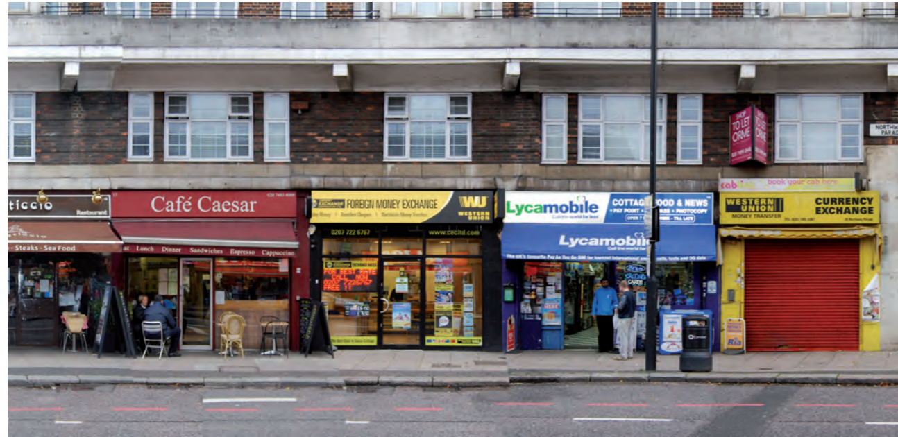
E6. Existing shopfronts facing Finchley Road
