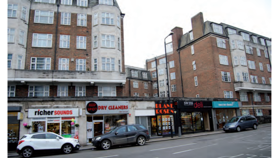
E4. Photograph of shopfronts facing College Crescent
