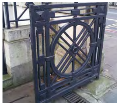
Existing listed gates retained
