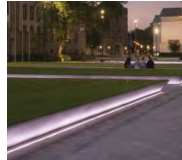
Integral LED strips to raised stone edges.
