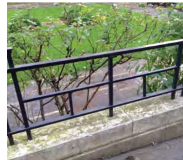
Existing listed railings retained
