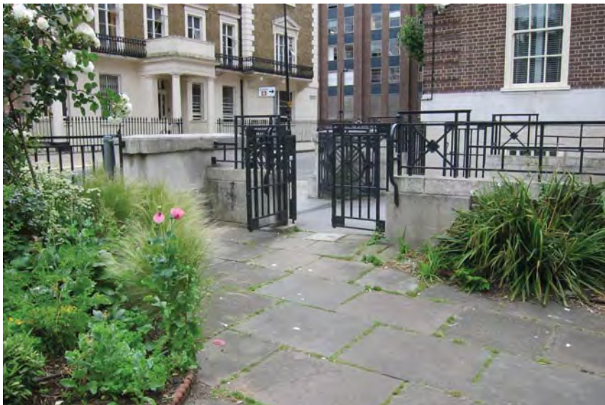
Balustrades and railings have heritage value but need coordination to make connections with the garden.
