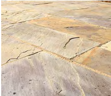
Reclaimed riven Yorkstone paving to terraces area and secondary footpaths.
