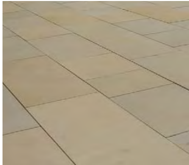
New Scoutmoor Yorkstone paving, random sizes to main pedestrian areas.
