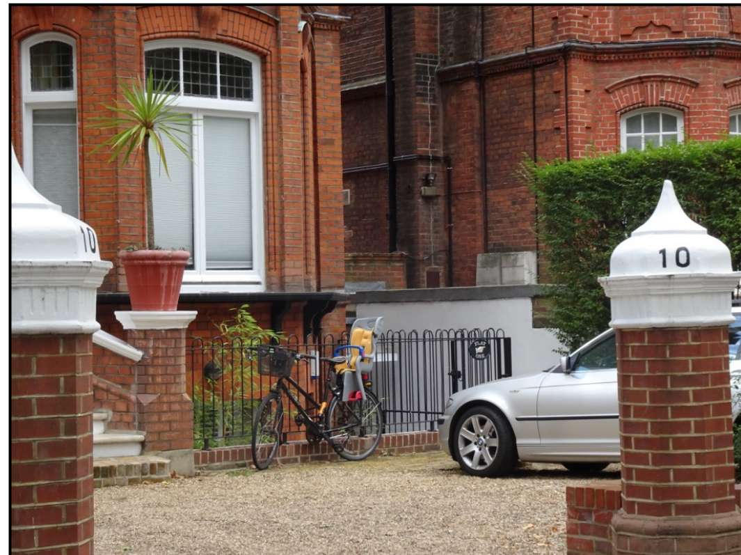
PHOTO C (Existing front elevation to 10 Strathray Gardens showing existing metal railings to basement)
