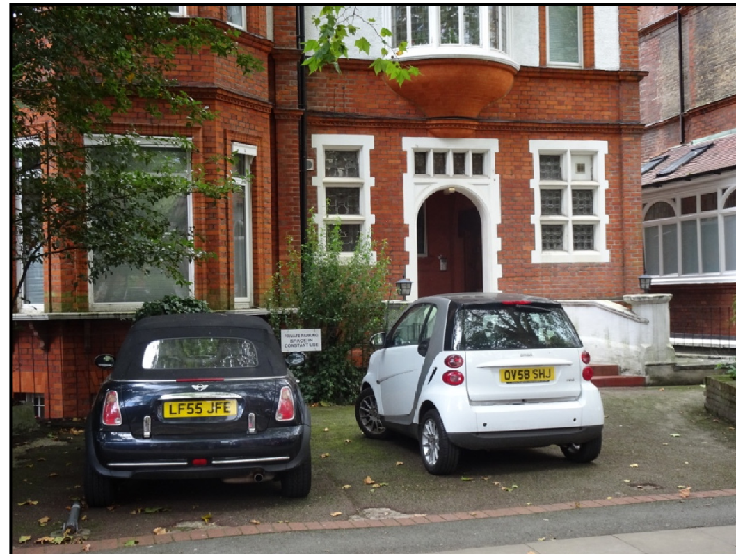
PHOTO D (Existing front elevation to 12 Strathray Gardens showing existing metal railings to basement)
