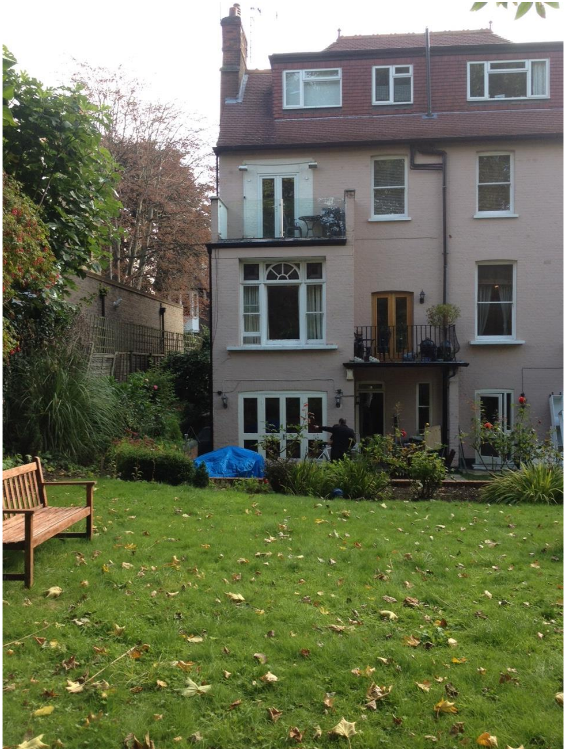
Photo 2- Rear elevation of subject site
