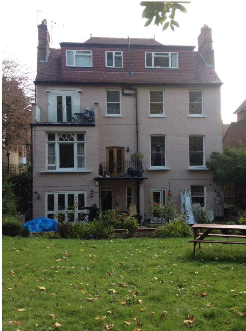
Photo 1- Rear elevation of subject site
