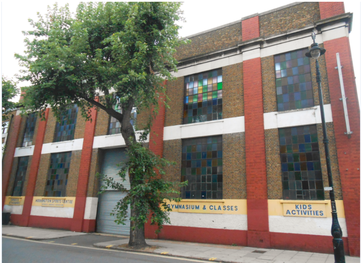
Photo 1: Western front elevation of the building
