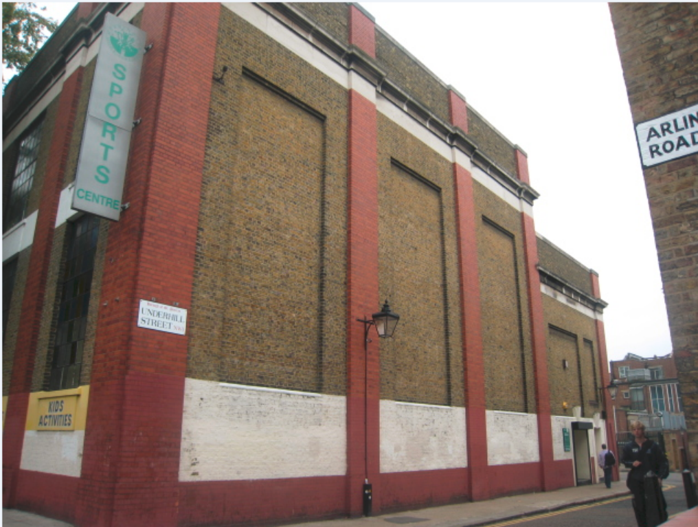
Photo 2: Southern side elevation of the building
