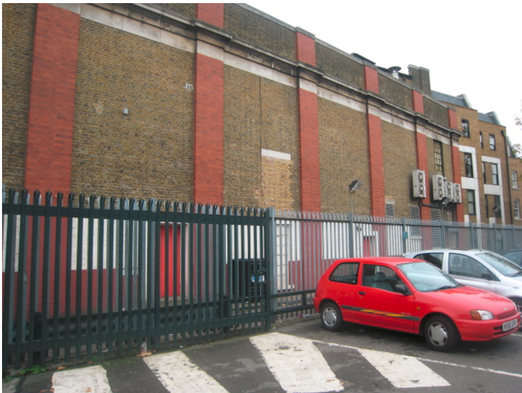
Photo 3: Eastern rear elevation of the building
