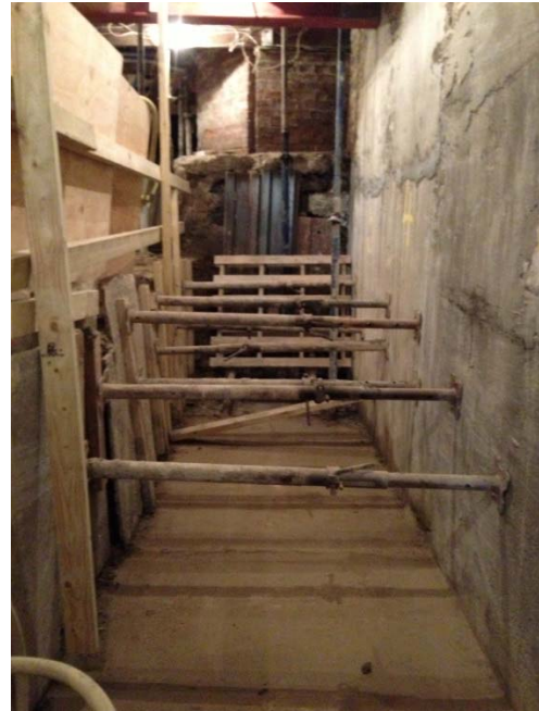
Image of Stage 3 on Site
