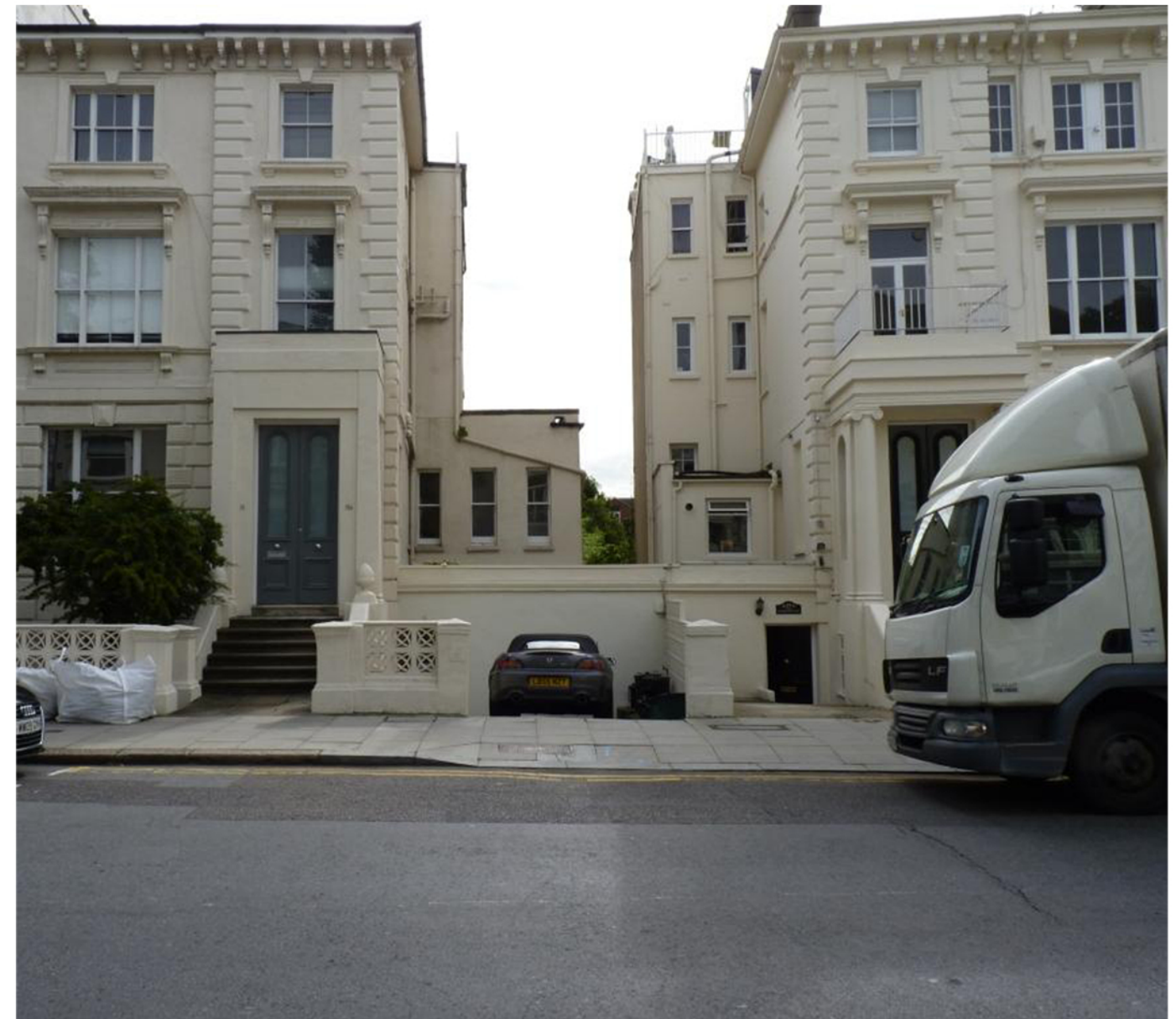
GENERAL VIEW OF 15 BUCKLAND CRESCENT
