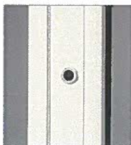
Flush lock with ferrule
