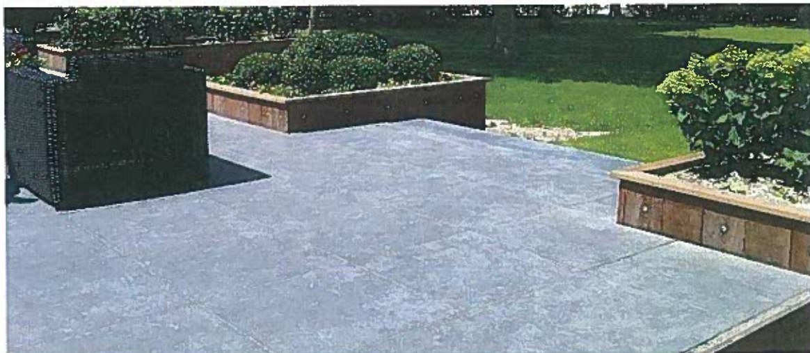
Weatherproof and lightweight 20 mm thick and load bearing Porcelain tiles for outdoor use
