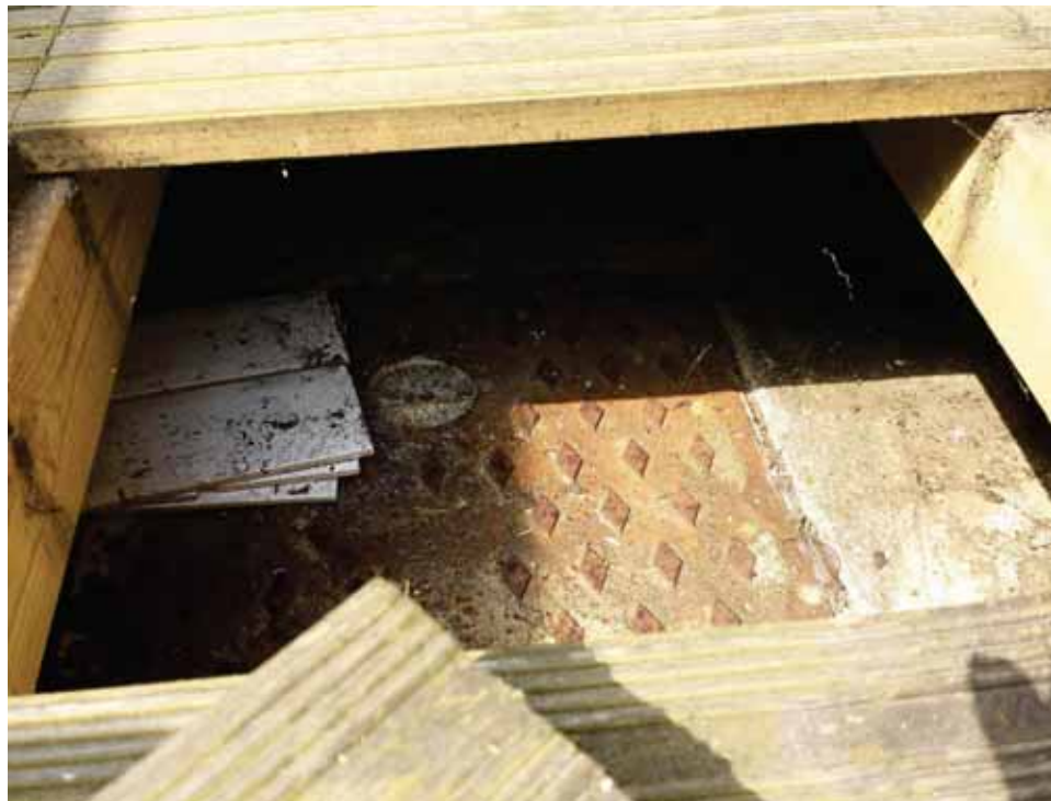
Figure 29: manhole in the rear garden
