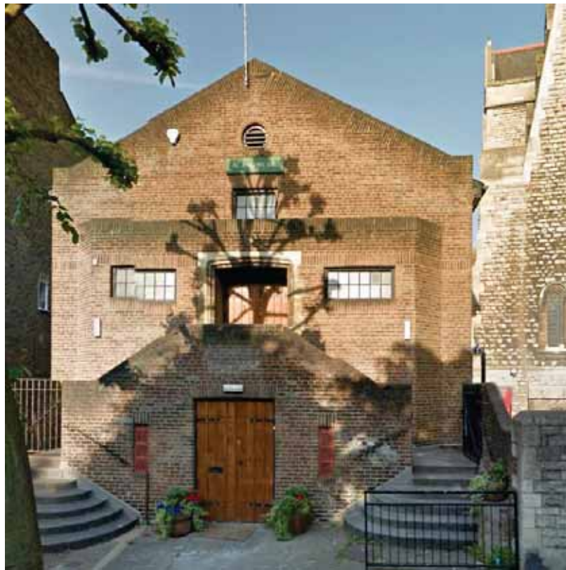
Figure 22: Front elevation of No. 53 Courthope Road
