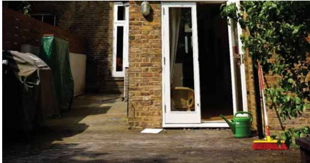
Figure 31: Existing hardstanding in the rear garden
