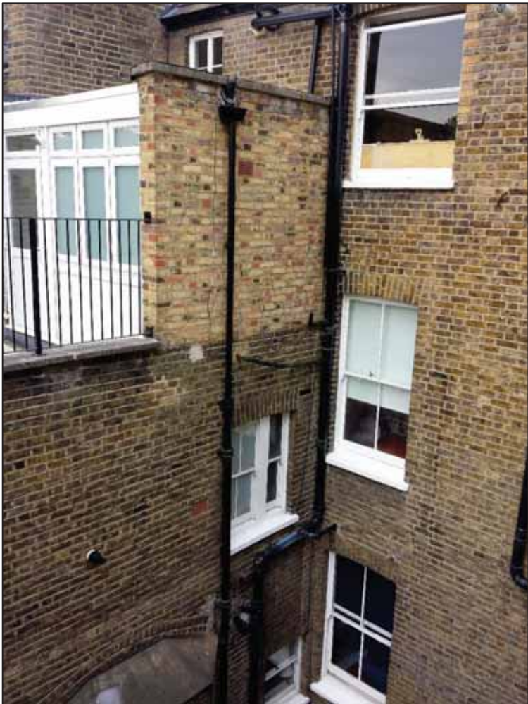
Figure 21: Rear wall of No 52 Shirlock Road
