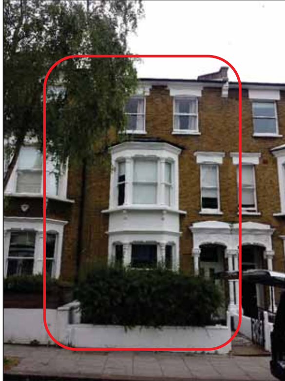
Figure 18: Front elevation of 52 Shirlock Road
