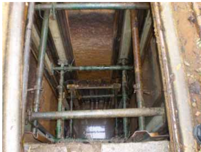
Figure 34 Propping
