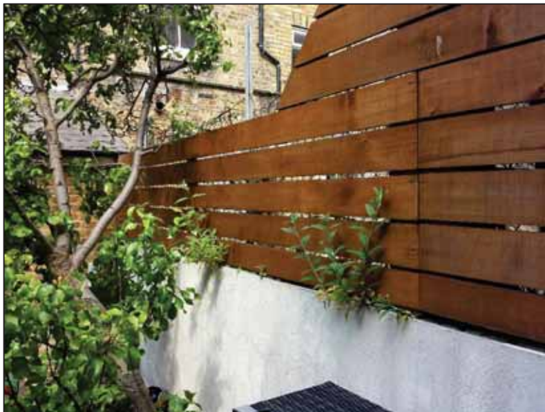
Figure 17: Boundary garden wall between 54 and 56 Shirlock Road
