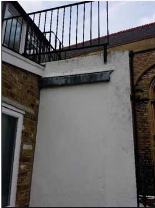
Figure 16: Rear roof terrace party wall
