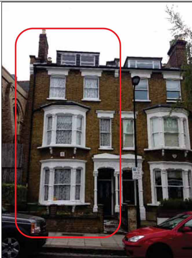
Figure 14: Front elevation of 56 Shirlock Road
