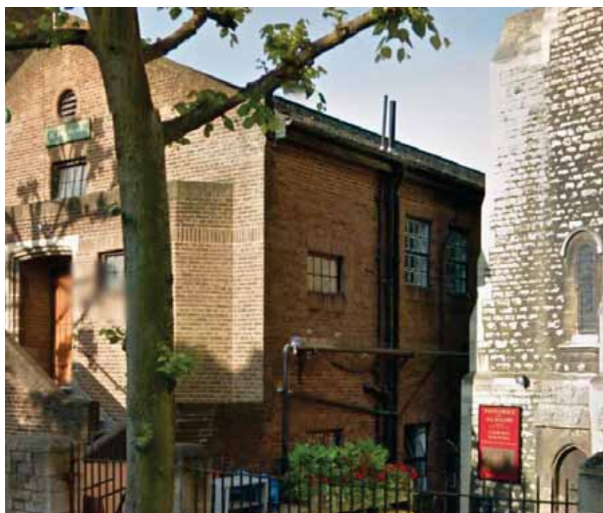
Figure 24: Right hand side wall of No 53 Courthope Road
