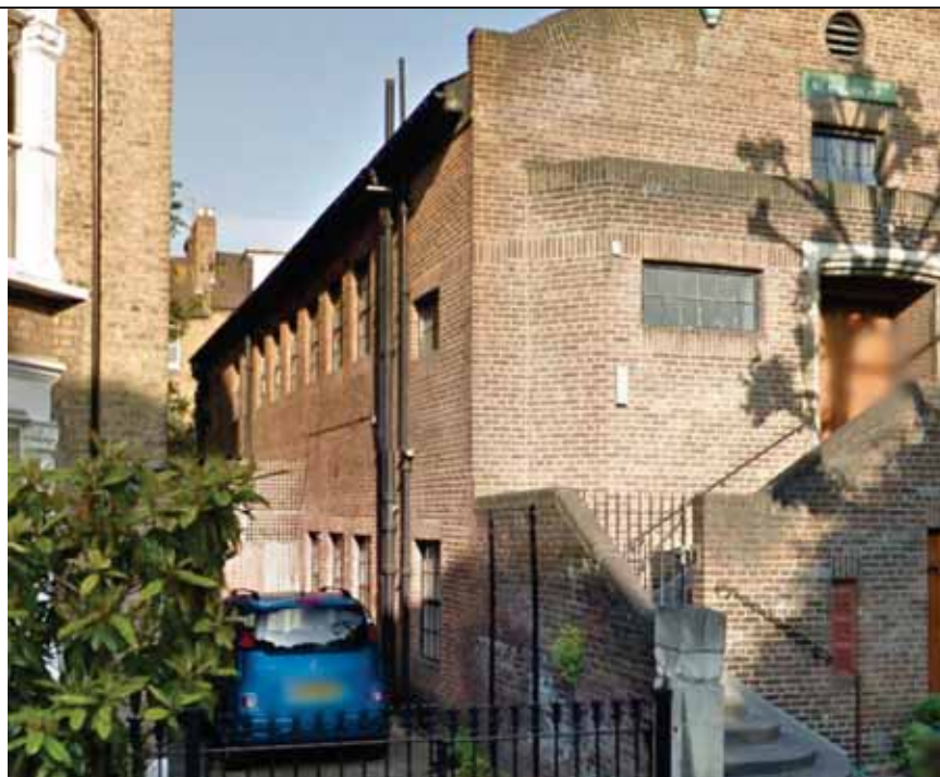
Figure 23: Left hand side wall view of No 53 Courthope Road
