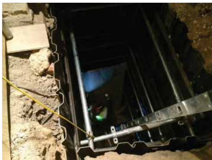
Figure 35 Excavation of Pin
