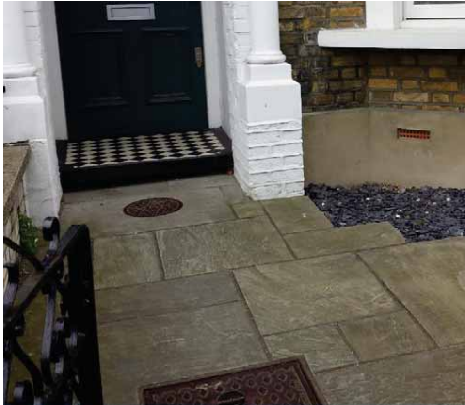
Figure 28: Front yard manholes
