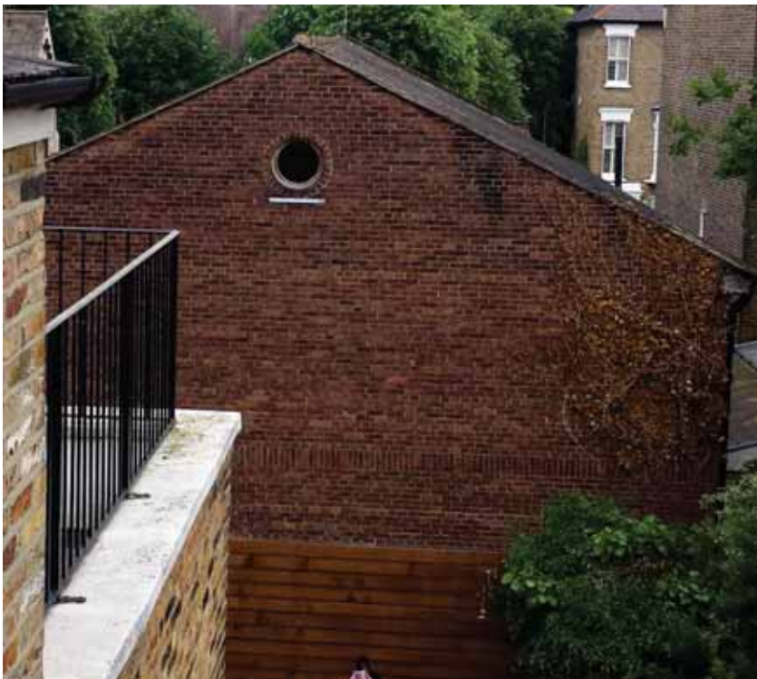
Figure 25: Rear views of 53 Courthope Road
