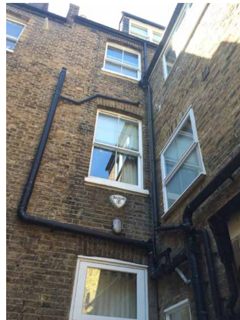
Side elevation view of the rear closet wing showing the largely reconstructed brickwork, modern window openings and window frames. Main body of house remains largely as built.
