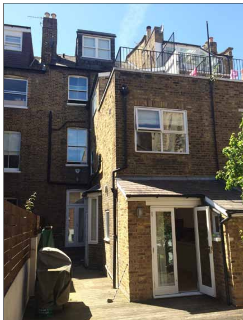
View of rear of house showing first floor arrangements to the rear facade of the existing closet wing. This element of the house has been largely reconstructed with a modern shaped opening with modern window design along with modern concrete coping and railings above.
