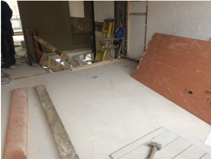
second floor screed
