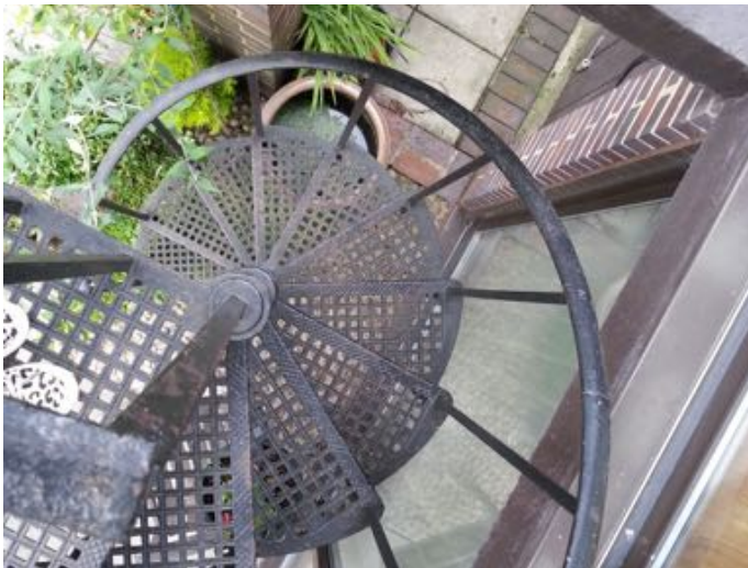
spiral stair to rear balcony
