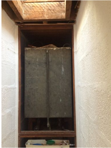
second floor rear of shower room
