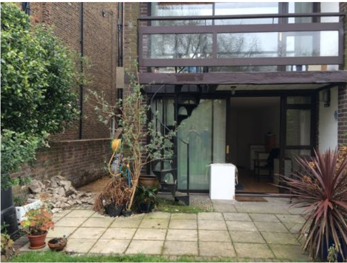
side extension demolished
