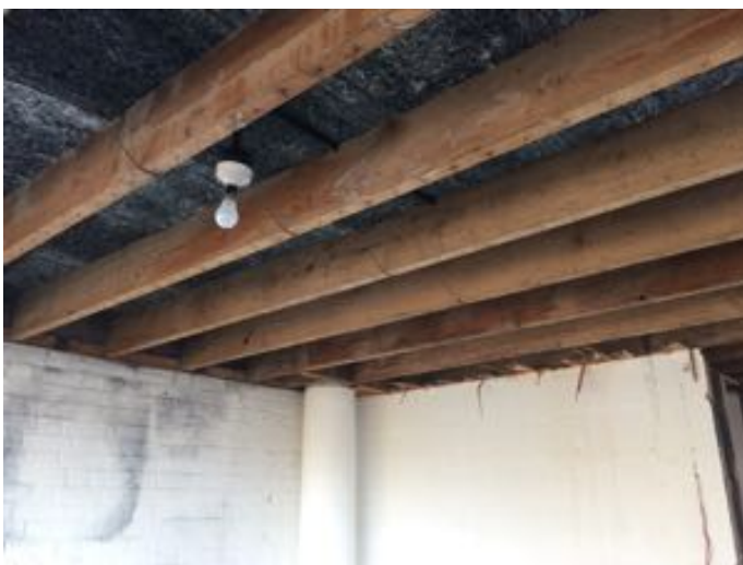
second floor roof structure from beneath
