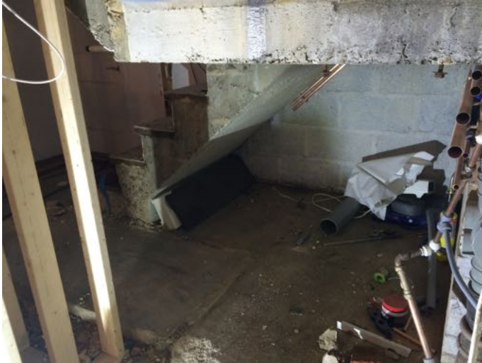
existing reinforced concrete stairs
