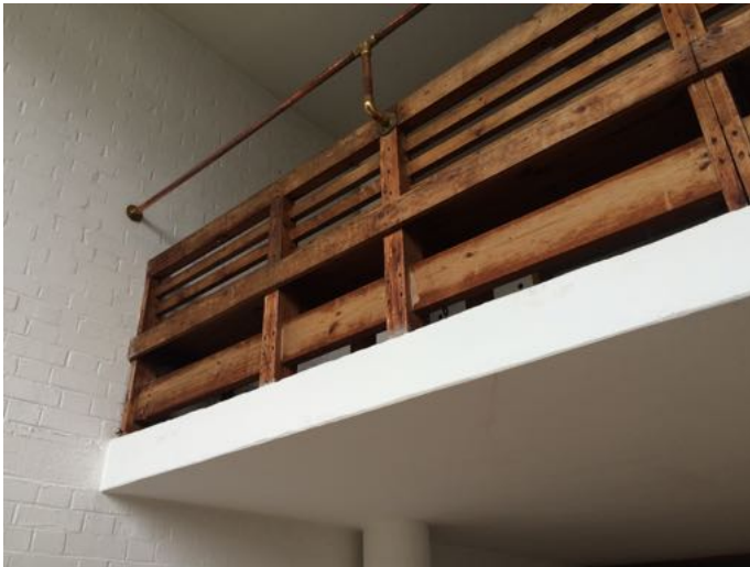
living room/mezzanine timber bench with copy handrail
