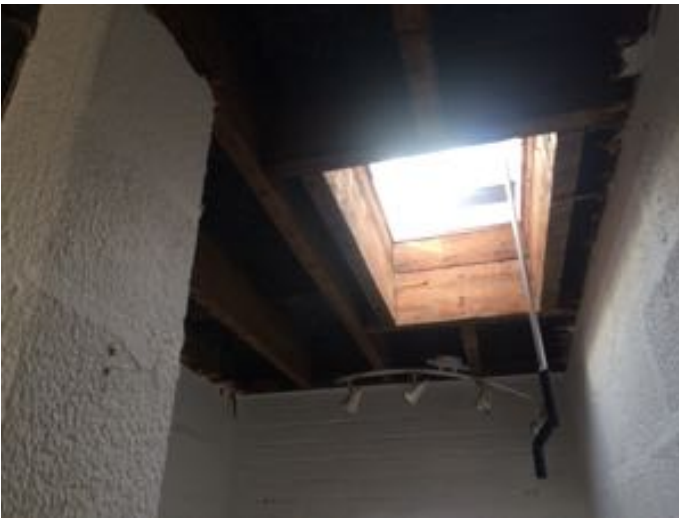
bathroom roof light
