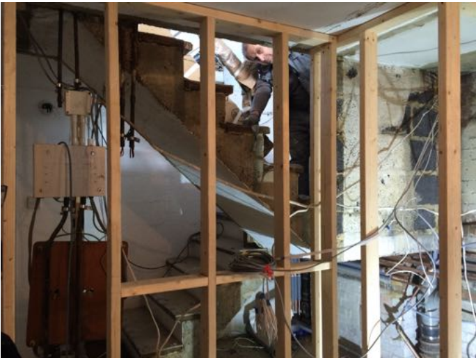
timber framing to new plant area
