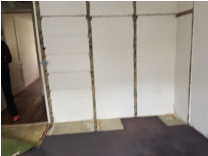
first floor living room
