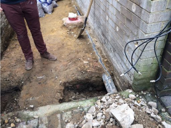
ground works to side of building
