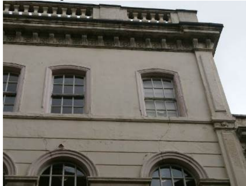
Right Hand Side Elevation – Second & First Floor - flaking decoration and cracking at window heads.
