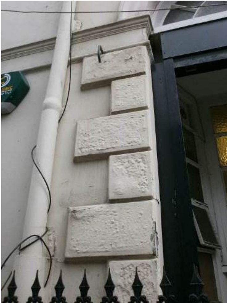
Right Hand Side Elevation - Flaking decorations. Paint-obscured vermiculated render panels.
