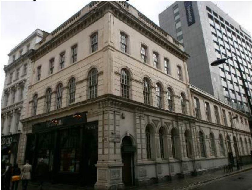
Front Right Hand Corner - flaking decoration. Paint-obscured vermiculated render panels.
