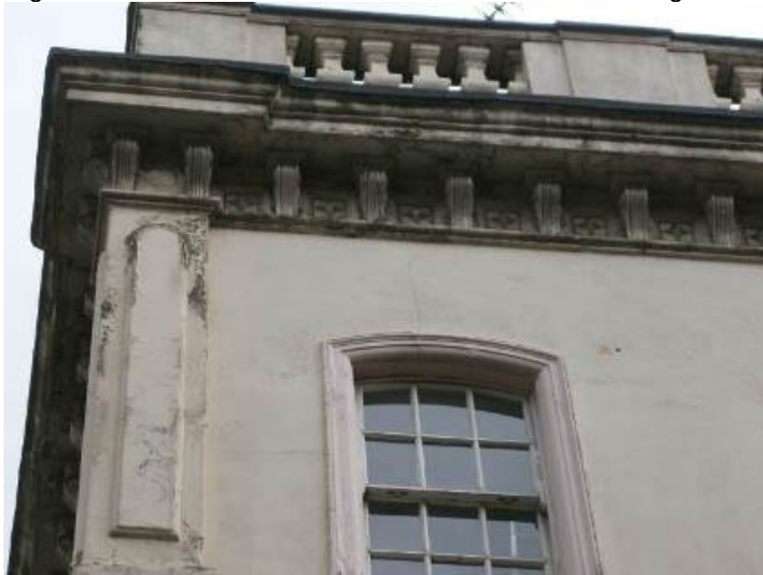
Right Hand Side Elevation – Second & First Floor - flaking decoration and cracking at window heads.
