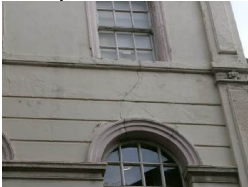
Right Hand Side Elevation – First & Ground Floor - flaking decoration and cracking at window heads.
