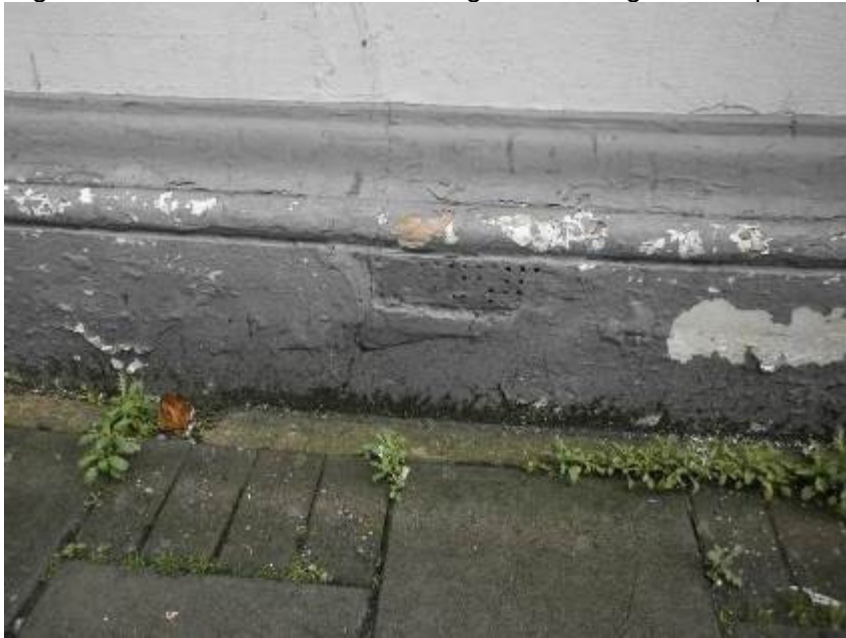
Right Hand Side Elevation - cracking and weed growth to plinth. Flaking decorations. Paint-obscured vermiculated render panels.
