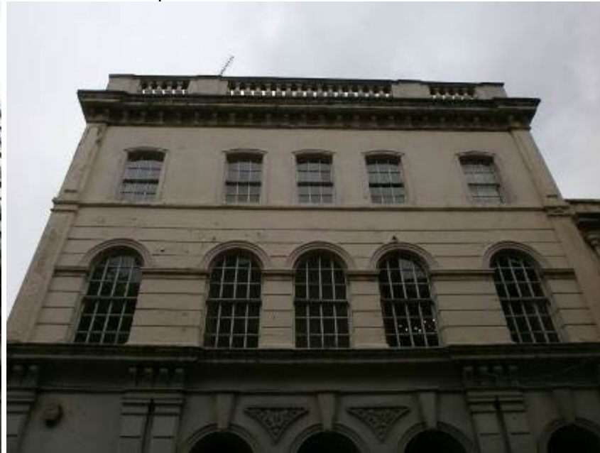
Front Right Hand Corner - flaking decoration. Paint-obscured vermiculated render panels.
