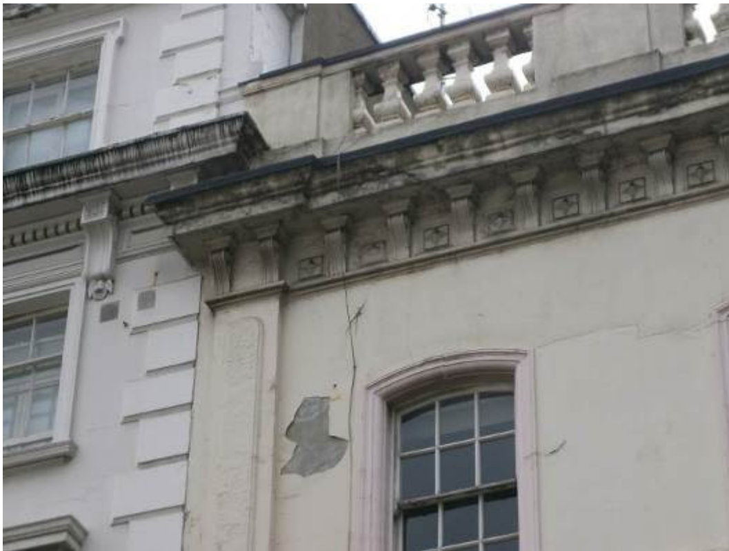
Front Elevation – Second Floor left hand side – flaking decoration & cement render
