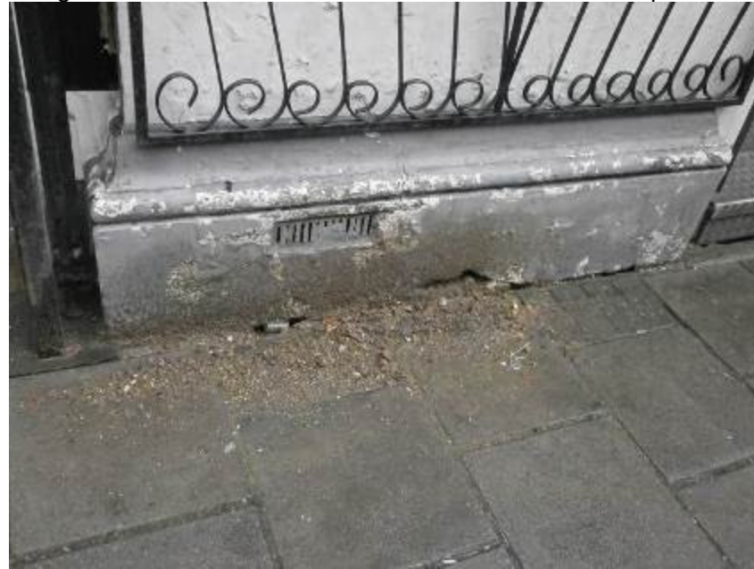
Right Hand Side Elevation - cracking and weed growth to plinth. Flaking decorations. Paint-obscured vermiculated render panels.
