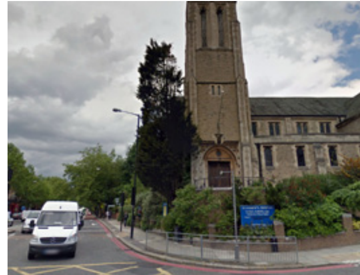
3. View from the junction of Froggnal Lane
