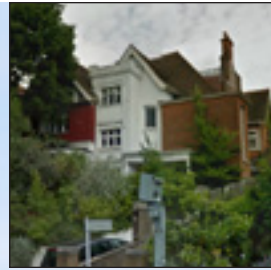
252 FINCHELY ROAD Neighbouring the church is an existing residential.
