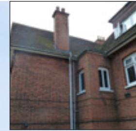
254 FINCHELY ROAD A stand alone building current use of residential apartments.
