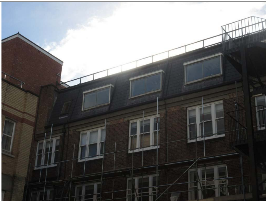
18: Rear elevation - existing aluminium sliding windows to 4 th floor mansard roof
