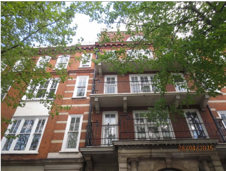
06: Front elevation – timber sliding sash windows to 1 st , 2 nd and 3 rd floors
