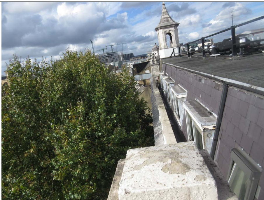
08: Front elevation – existing aluminium sliding windows to 4 th floor mansard situated behind parapet wall
