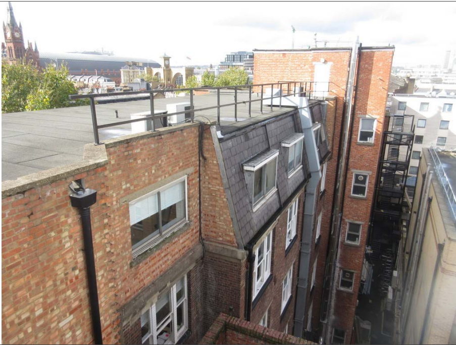
21: Rear elevation - existing aluminium sliding windows to 4 th floor mansard roof
