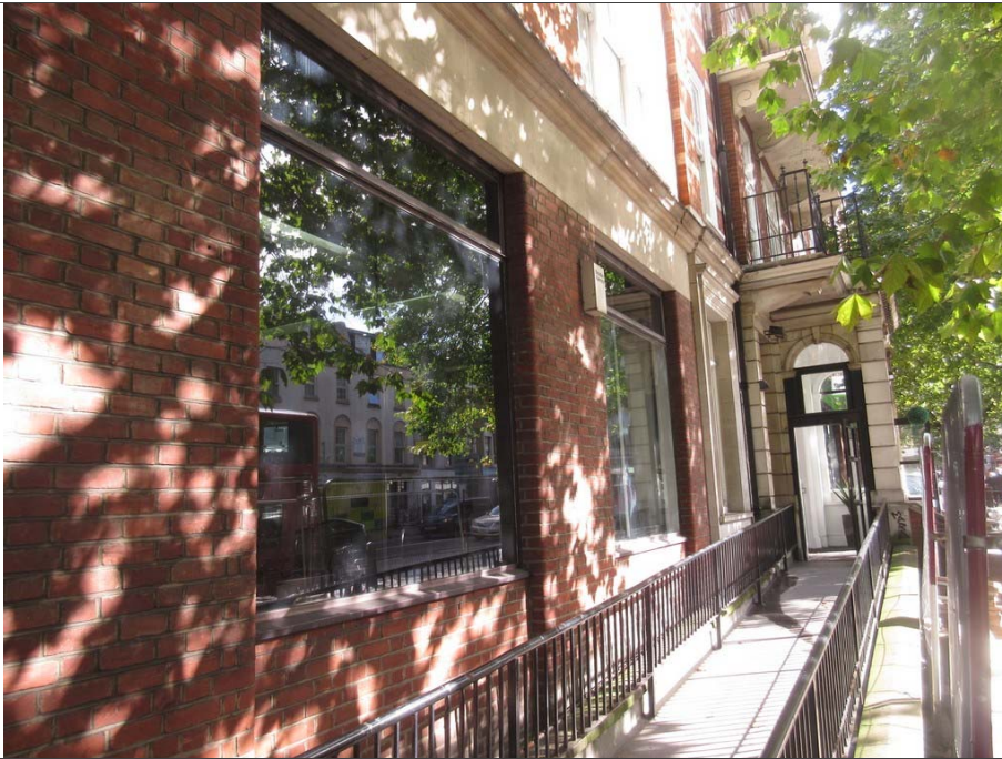
05: Front elevation – powder coated aluminium windows to ground floor
