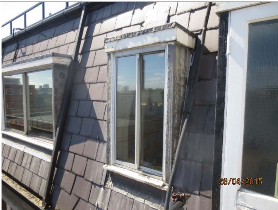
20: Rear elevation - existing aluminium sliding windows to 4 th floor mansard roof
