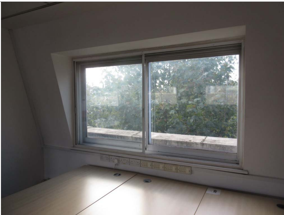
22: Front elevation – internal view of existing sliding windows to 4 th floor with secondary glazing
