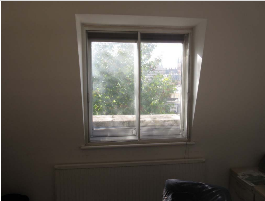
23: Front elevation – internal view of existing sliding windows to 4 th floor with secondary glazing
