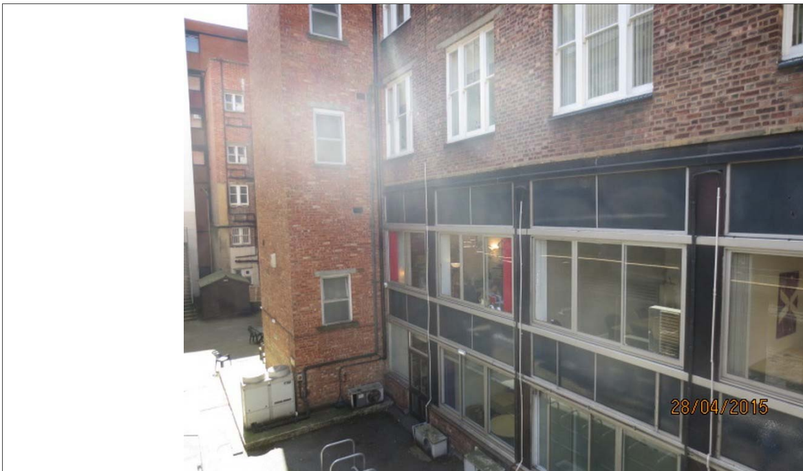
16: Rear elevation - metal framed windows to lower ground and ground floors
