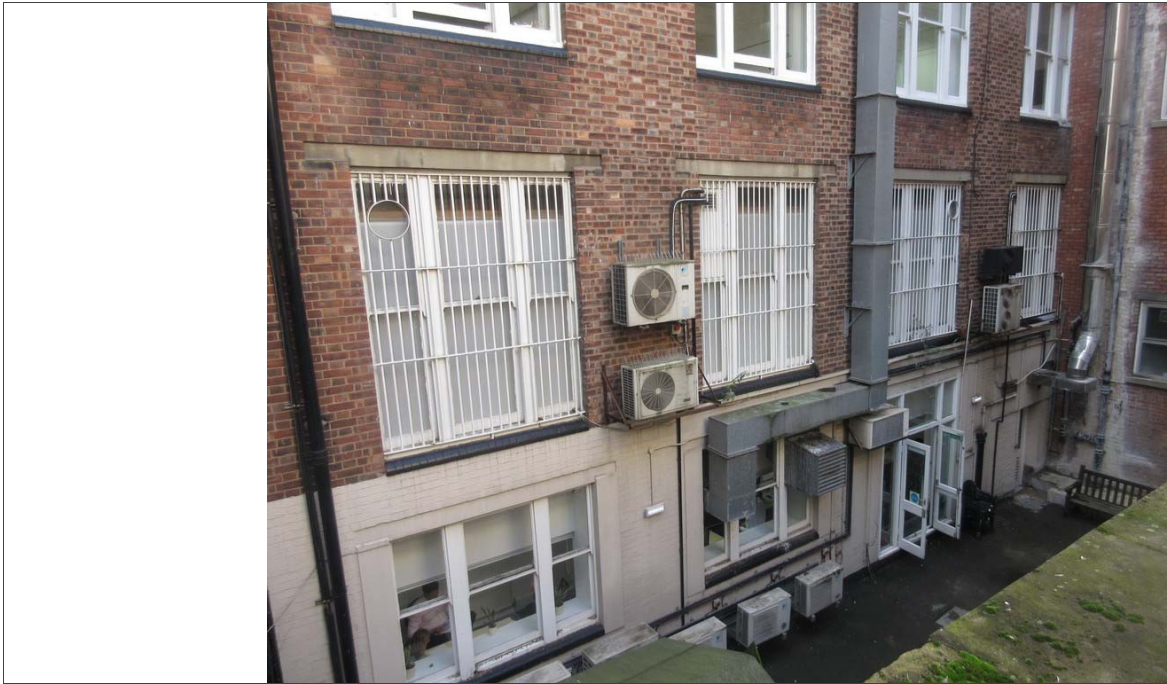
13: Rear elevation - timber sliding sash windows to lower ground and ground floors
