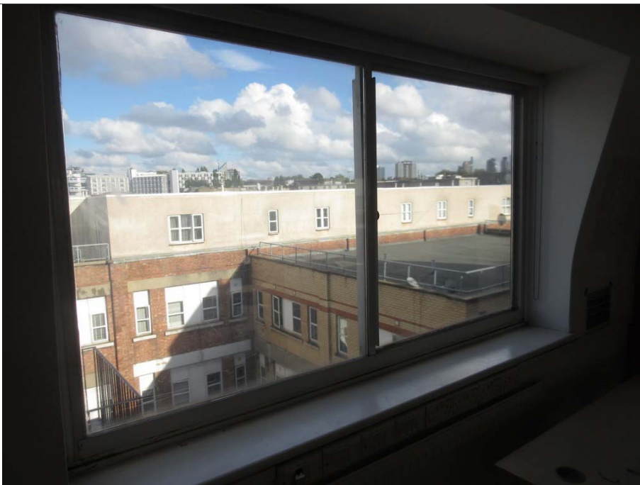
24: Rear elevation – internal view of existing sliding windows to 4 th floor
