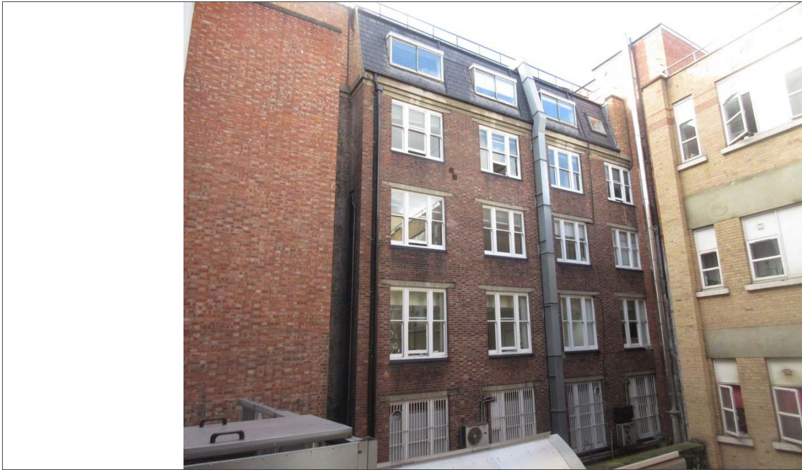
15: Rear elevation - timber sliding sash windows to ground, 1 st , 2 nd and 3 rd floors
