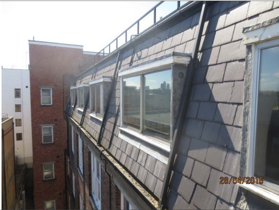
19: Rear elevation - existing aluminium sliding windows to 4 th floor mansard roof
