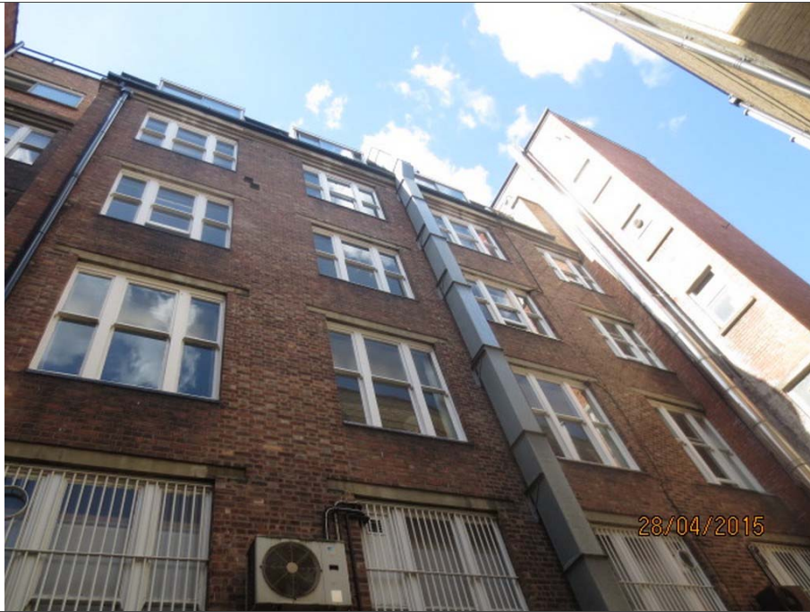
17: Rear elevation - timber sliding sash windows to ground, 1 st , 2 nd and 3 rd floors
