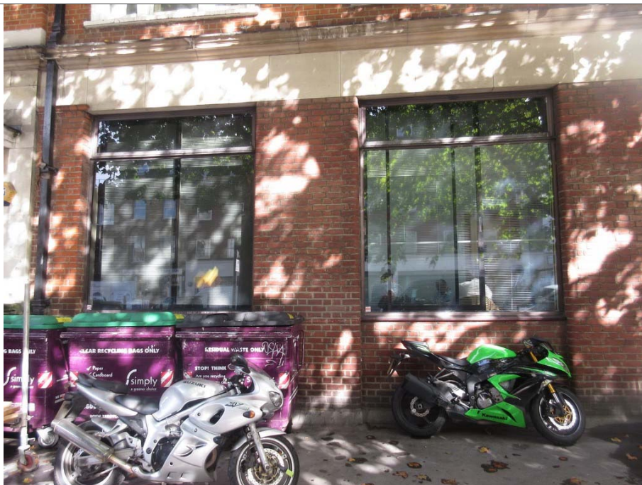
04: Front elevation – powder coated aluminium windows to ground floor
