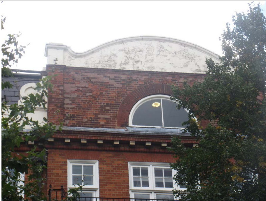
11: Front elevation – frost shattered brickwork below rendering and around semi circular window
