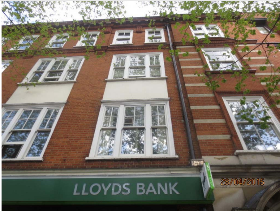
07: Front elevation – timber sliding sash windows to 1 st , 2 nd and 3 rd floors
