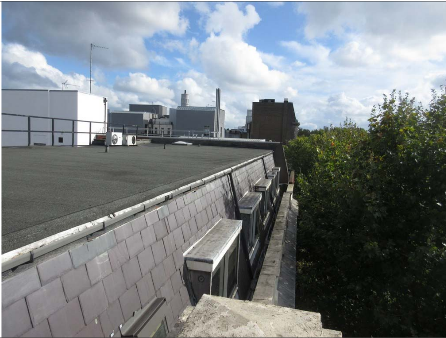
09: Front elevation – existing aluminium sliding windows to 4 th floor situated behind parapet wall
