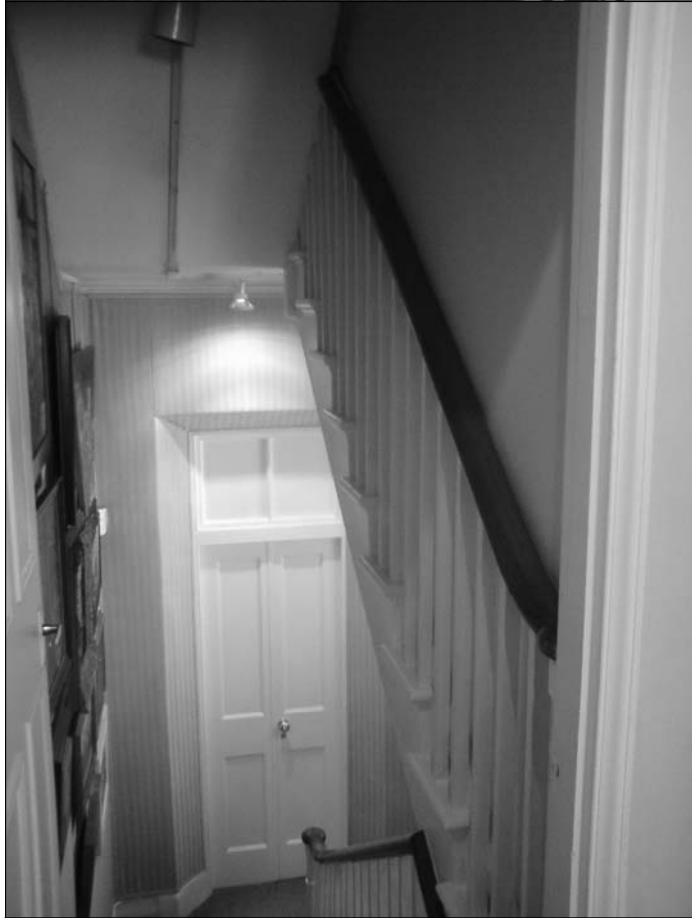
S5 STAIRCASE PARTITION REMOVED TO REVEAL ORIGINAL HANDRAIL AND BALUSTRADE
