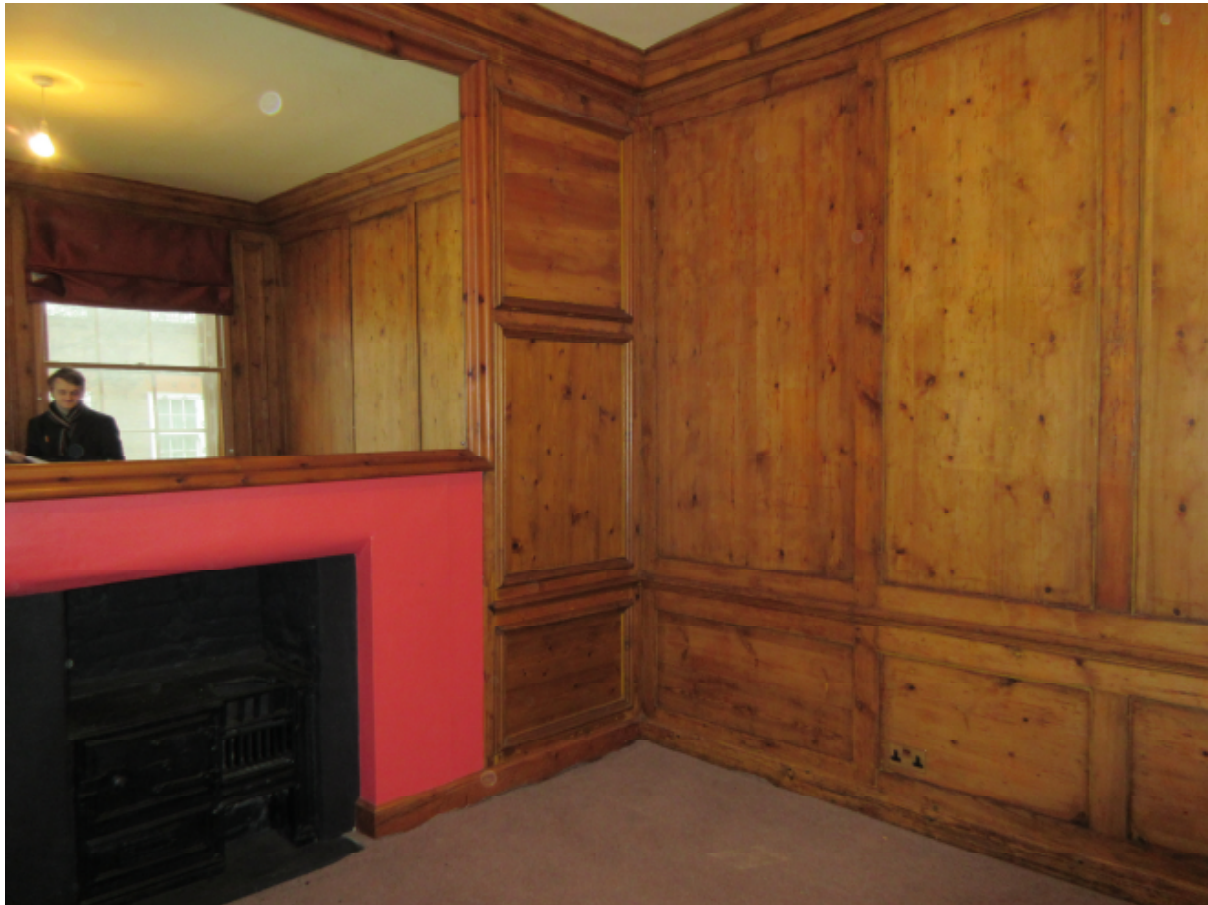
Picture 6: first-floor east front room. Note brand-new cooking stove in fireplace – clearly not an original feature of the piano nobile of a grand townhouse. To be replaced with suitable fireplace. Panelling to be repaired and matched where missing.
