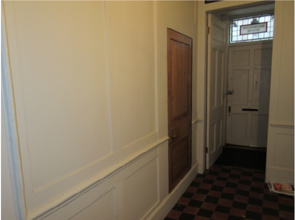
Picture 2: the entrance hall. Note blocked door to be reopened. The non-historic pocket door to right will be replaced to match this door in style. Non-historic storm porch will move to fit better with panelling.
