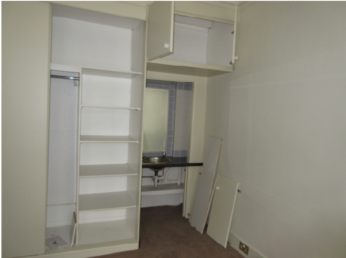
Picture 13: second-floor east front room, alcove to be reinstated as doorway – partition is made of modern plasterboard and stud partition.
