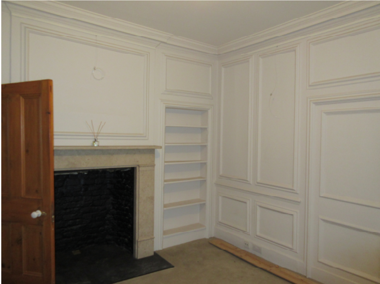
Picture 3: ground-floor front room. Non-original fireplace to be replaced with suitable, smaller surround to be in proportion with room. Non-original bookshelf/alcove to become doorway. Original architrave indicates original presence of doorway to be reinstated to balance doorway on left.
