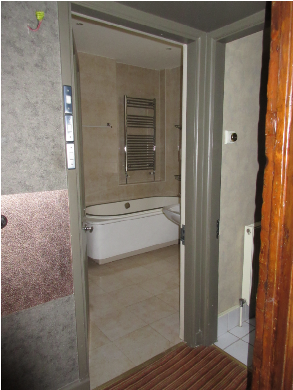
Picture 10: second-floor rear west, modern bathroom off master bedroom; modern partition (with three switches) to be removed to reinstate original plan form of room.
