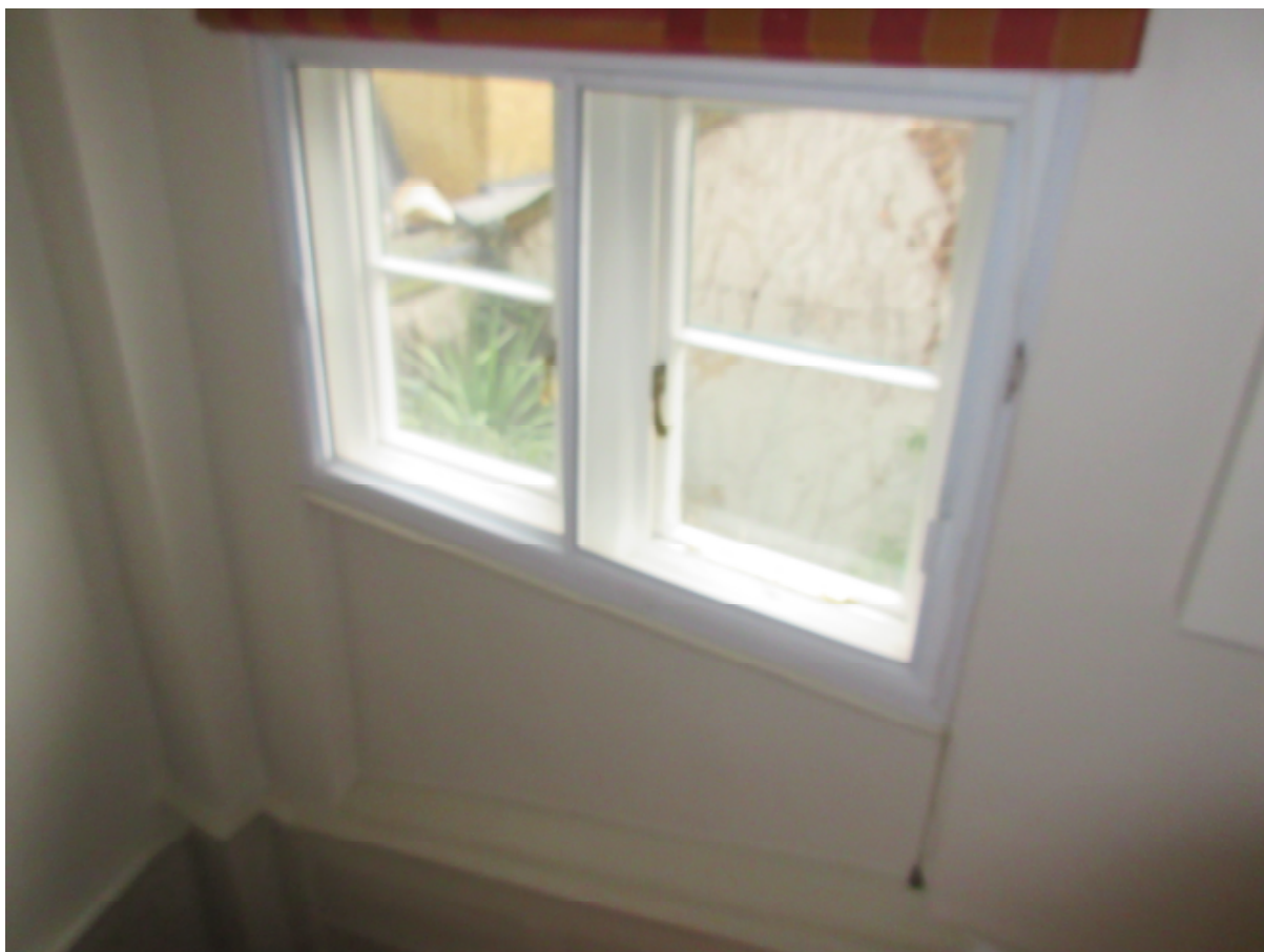
Picture 9: evidence of original shape of rear window. Non-original casement to be reinstated to sliding sash.
