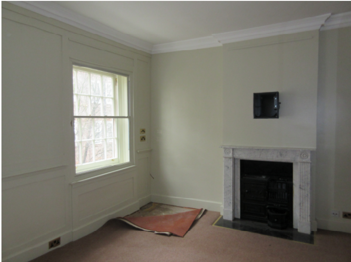
Picture 11: second-floor west front room, non-original fireplace in partially panelled second-floor room. Modest opening to be made through to master bathroom to right (out of shot) through modern plasterboard wall. Absent panelling to be supplied in differentiated MDF.
