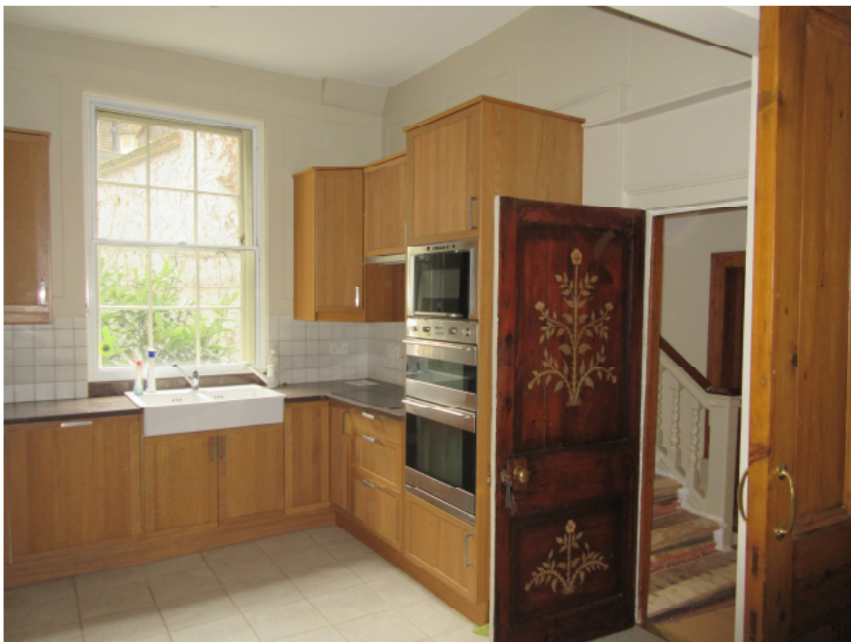
Picture 7: first-floor rear west room, currently configured as kitchen. Kitchen to be removed and existing panelling to be revealed. Surviving historic two-panel door to be used as pattern for rest of house, replacing Victorian six-panel doors.
