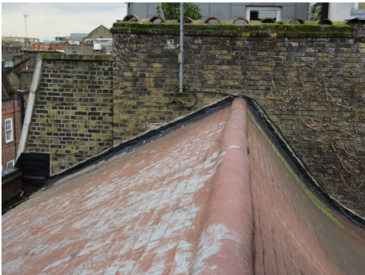
Picture 14: no alterations are proposed to roof but it has been coated in fibreglass. Applicant wishes to reinstate original pantiles like for like, salvaging any tiles that can be salvaged.
