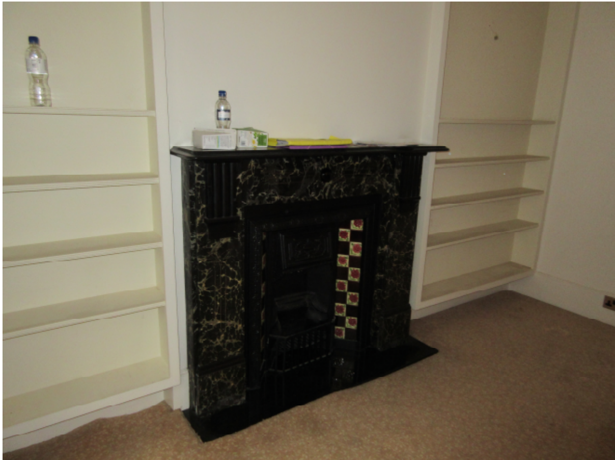
Picture 5: ground-floor western front room, non-original disproportionate fireplace to be removed and replaced with suitable model, bookshelves to be removed. Room will be simple panelled in MDF, as it is not currently panelled.
