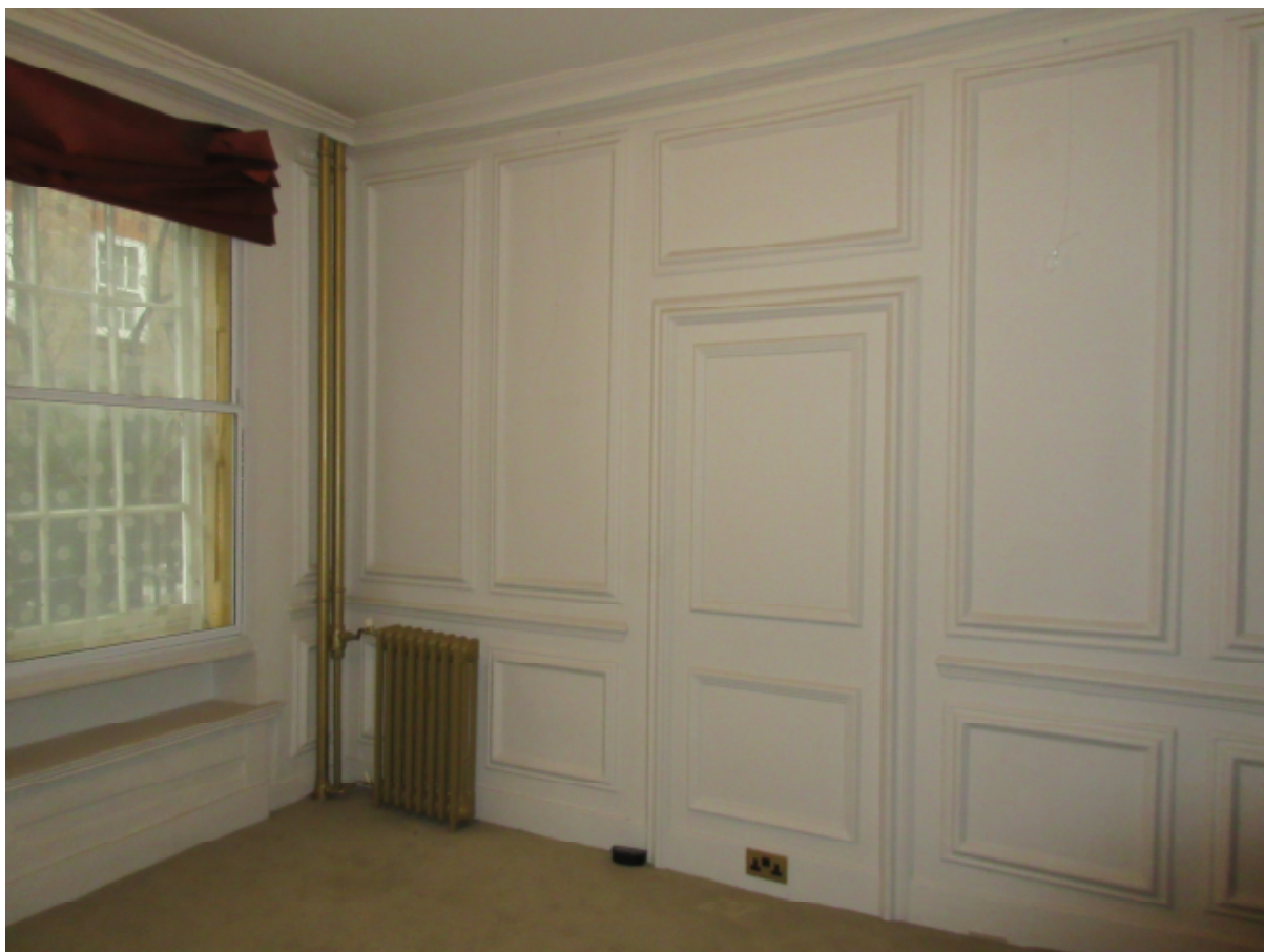
Picture 4: ground floor front room, reverse of blocked hall door to be reopened.
