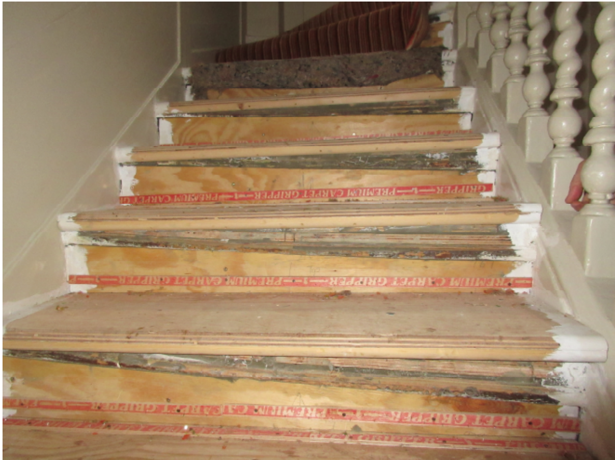
Picture 8: stairs have been heavily modified to level treads. Reinstatement in oak to be arranged by condition.
