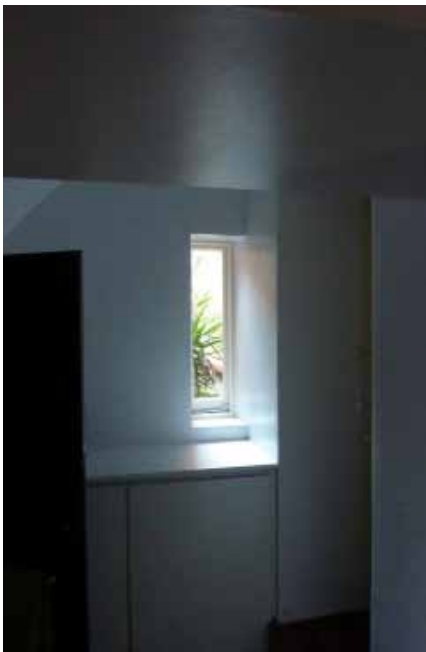
1_Replaced window inside
