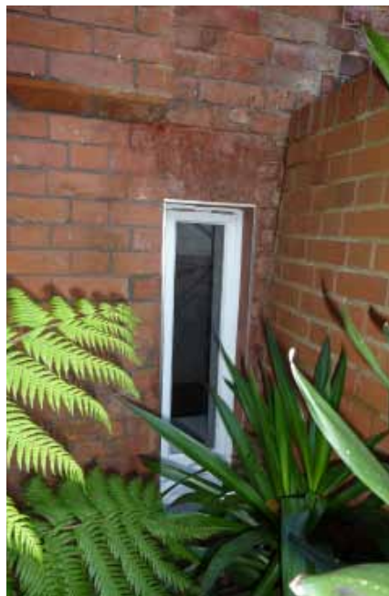
2_Replaced window outside
