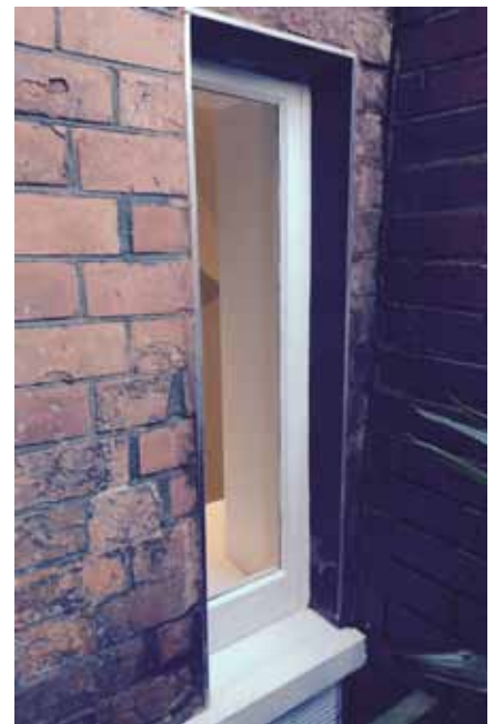
3_Replaced window outside
