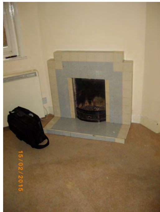
Fireplace in Rear Room 1 st Flr
