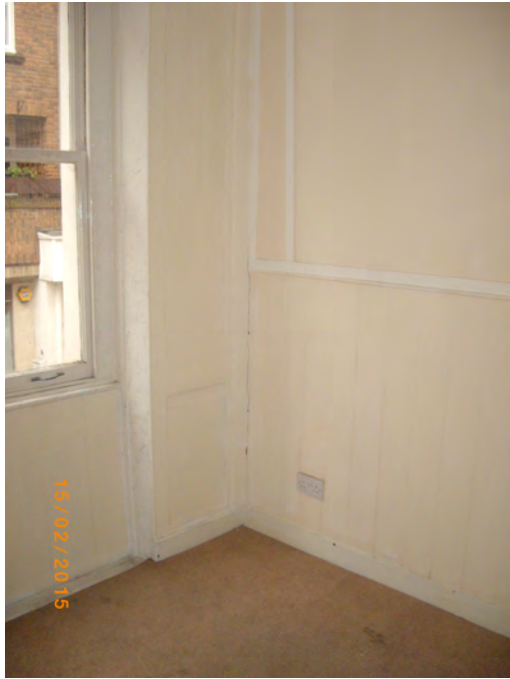
First Floor Front Room. Timber boarded to dado, panelling above
