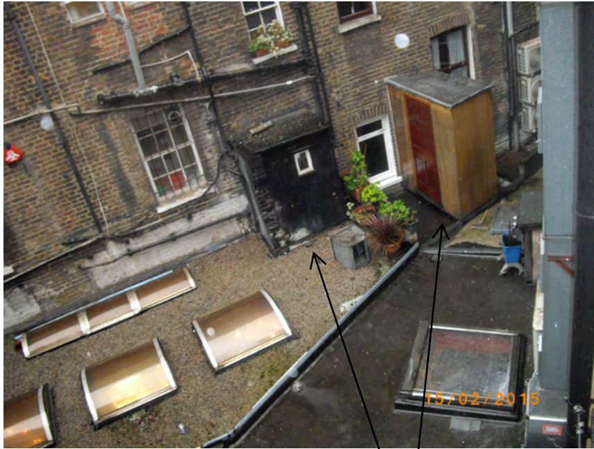
Minor extensions at 1 st floor level.
