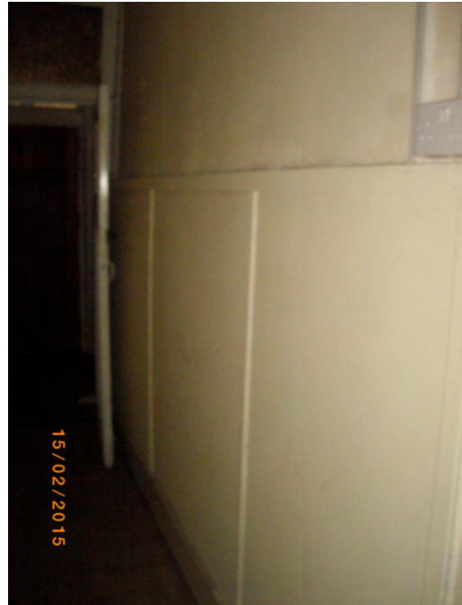
Front Hall access from Pavement
