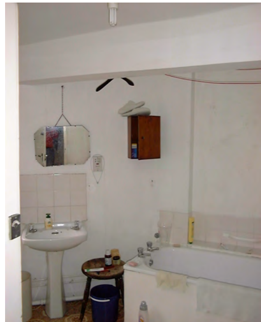
Original Drop Beam in 3 rd flr Bathroom. (Longitudinal)
