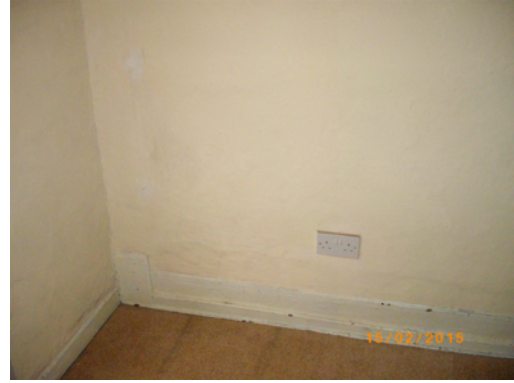
Originla skirting's and plaster. 2 nd Flr front room. No Panelling
