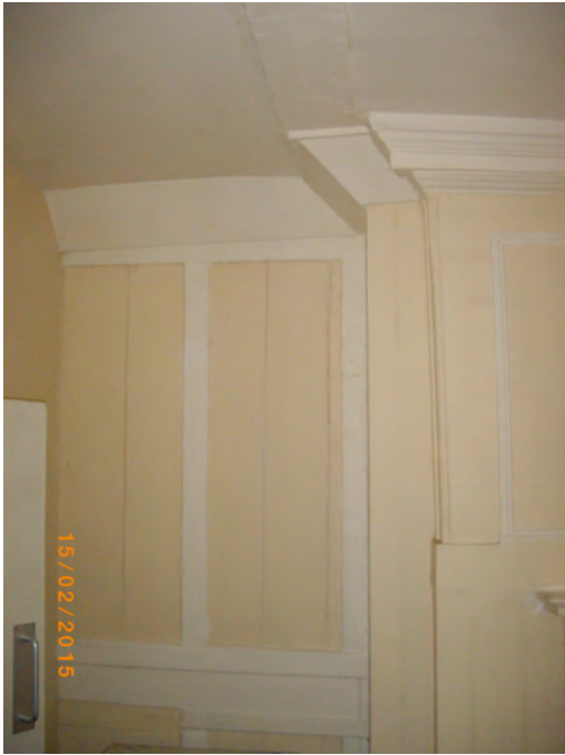
Panels above dado & Cornice 1 st Flr
