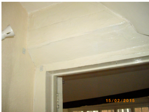
Original beam, transverse at 3 rd flr
