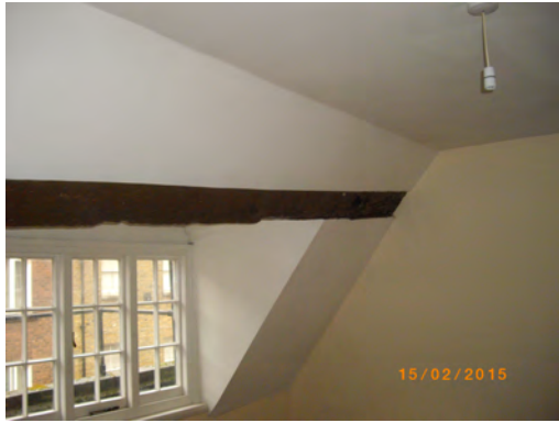
Original beam across Dormer At Third Floor
