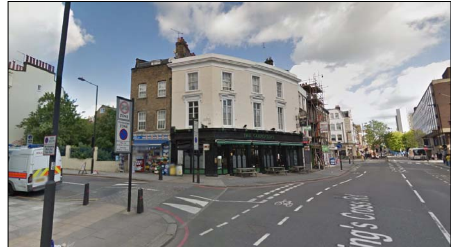
Fig 6. Existing Elevation along Frederick Street showing the adjacent building with a mansard.
