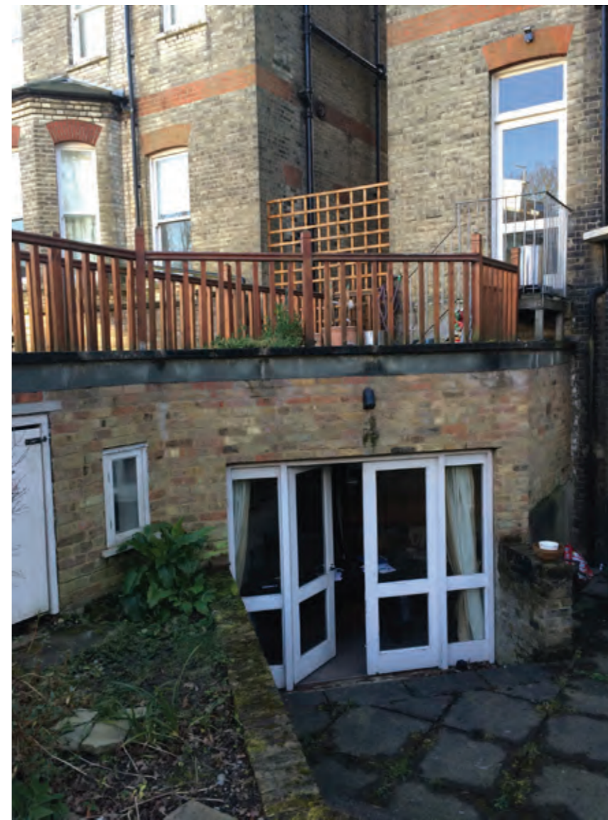
EXISTING REAR VIEW OF 21A CANNON PLACE
