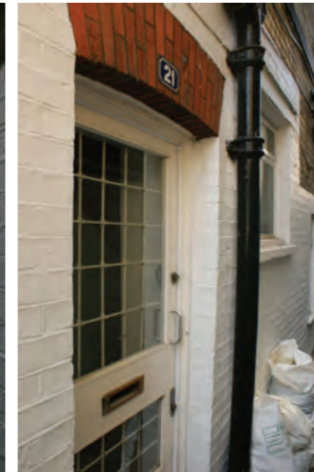
EXISTING ENTRANCE TO LOWER GROUND FLOOR LEVEL
