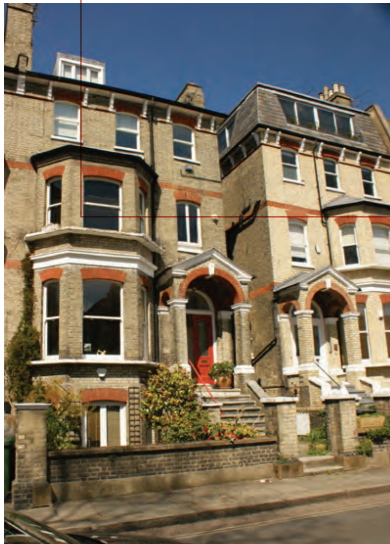
EXISTING FRONT VIEW OF 21A FROM CANNON PLACE
