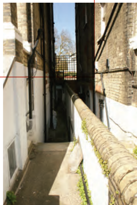
ACCESS TO 21A AT LOWER GROUND FLOOR LEVEL
