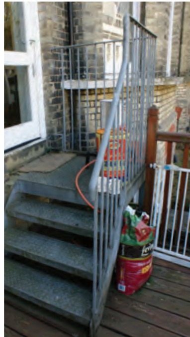
ACCESS TO TERRACE FROM KITCHEN
