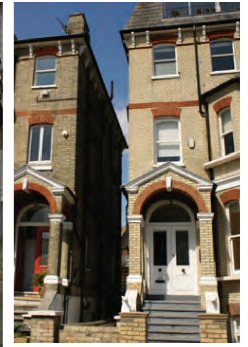
VIEW OF ALLEY ALONG EAST SIDE
