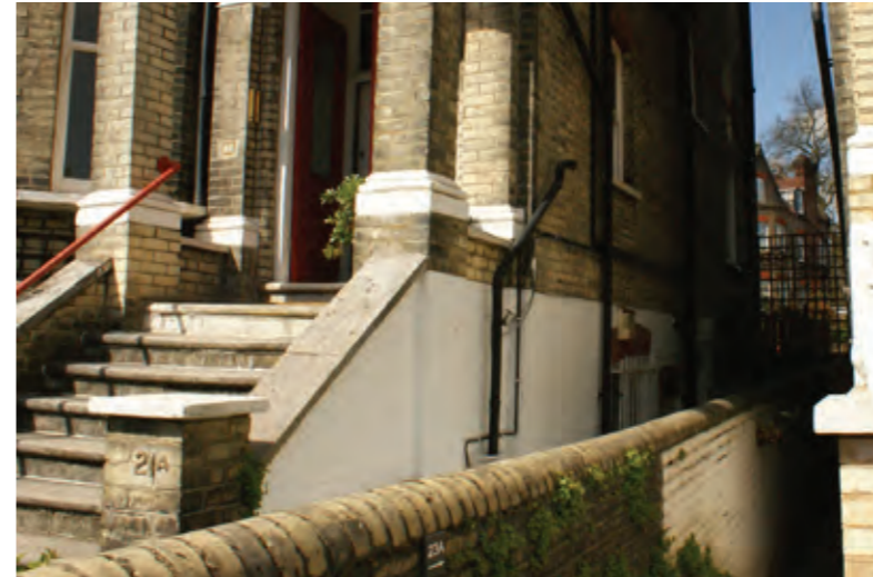
EXISTING BOUNDARY WALL AND EAST ELEVATION
