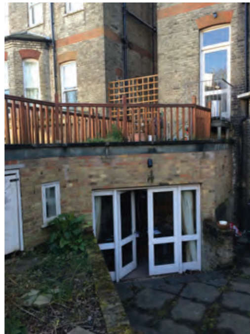
EXISTING STUDY ROOM DOORS TO THE 1975 REAR EXTENSION
