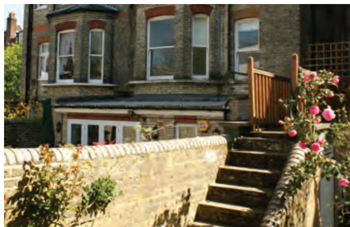
REAR GARDEN STEPS LEADING TO TERRACE
