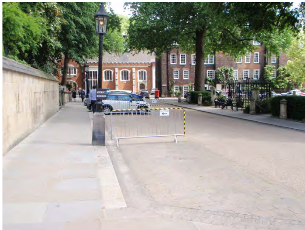
Figure 1.3: Existing Footway to South of Great Hall
