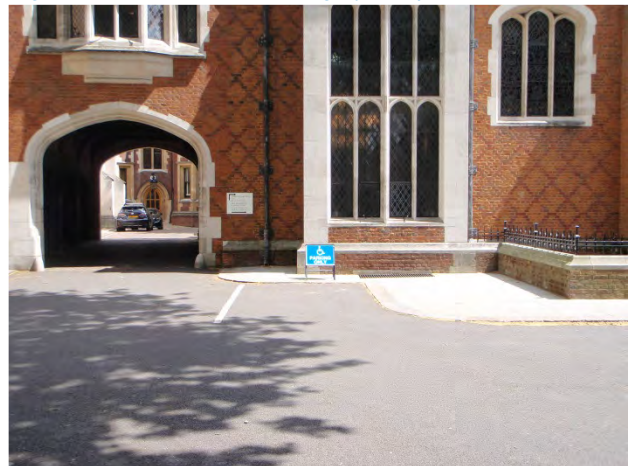
Figure 2.8: Disabled Parking by Chapel
