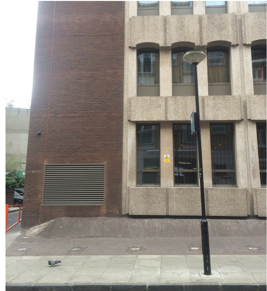
View of left side of site with ventilation grille and access to delivery service road.
