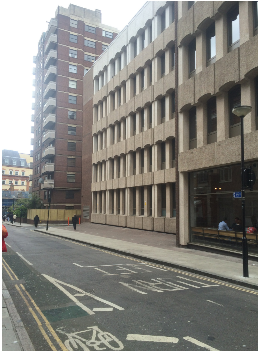
View of site showing retail unit on corner of High Holborn & Newton Street.
