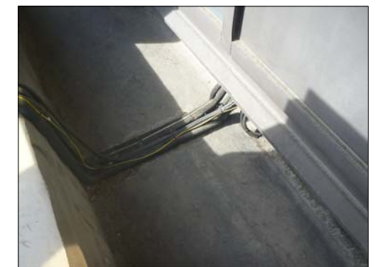
Survey photos of proposed location
