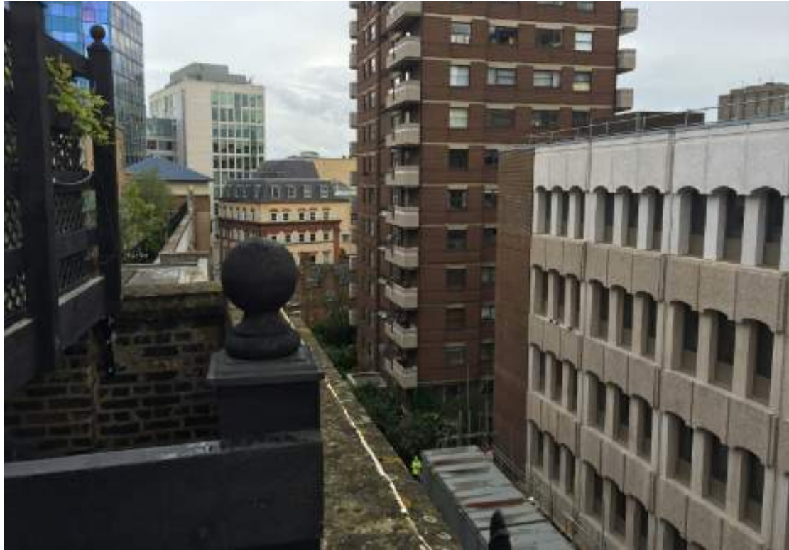
Photograph showing balustrading and setback from parapet on Newton Street (taken from entrance to roof terrace looking South)
