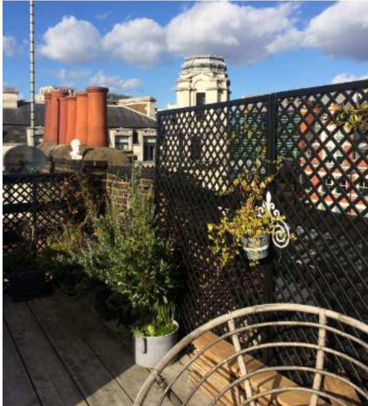
Photograph showing roof terrace with decking and balustrading (taken from the middle of the terrace looking North East)
