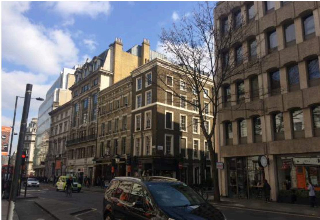
Medium distance view looking South East from High Holborn of the site at No. 207 High Holborn
