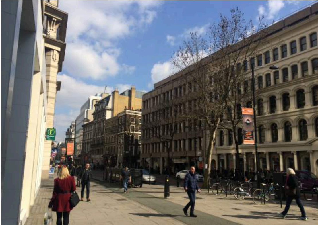
Long distance view looking South East from High Holborn of the site at No. 207 High Holborn
