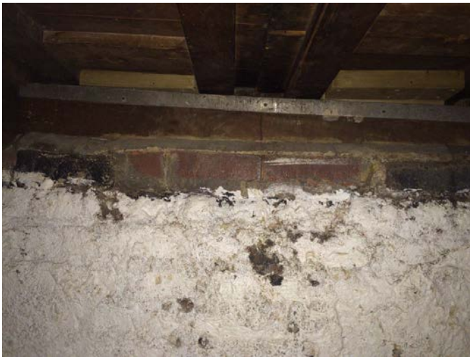
Photograph 3 – Internal view showing bricking up to line of internal cellar hatch
