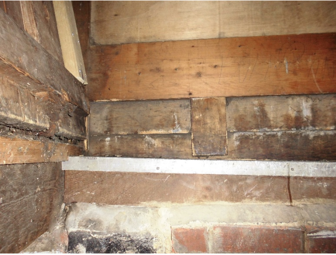
Photograph 5 – Detail of Internal Cellar Hatch
