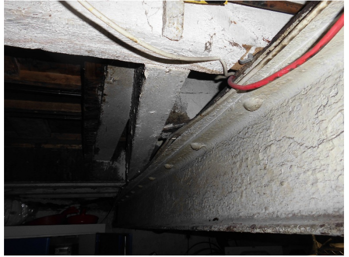
Photograph 6 – Framing around internal cellar hatch
