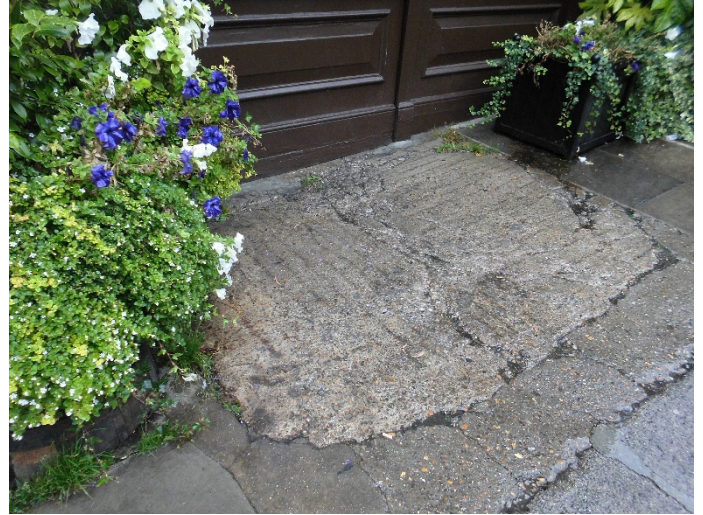
Photograph 2 – View of pavement adjacent in front of Woodsome Road elevation
