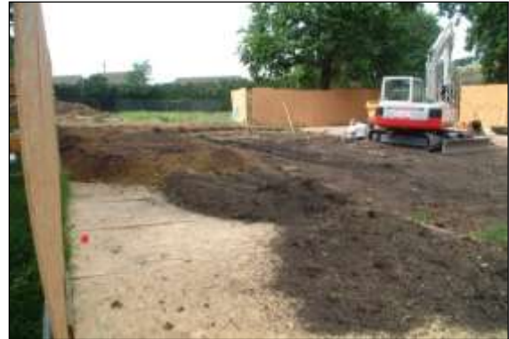
Photo 8: Spreading soil excavated from footings is an effective way of buffering the plywood surface from the wear of light vehicles.
