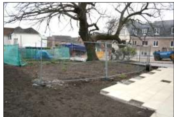
Photo 49: This tree had tarmac parking within its RPA that was removed and replaced with an organic mulch near the trunk and limited no-dig surfacing on the outer edges of its RPA.
