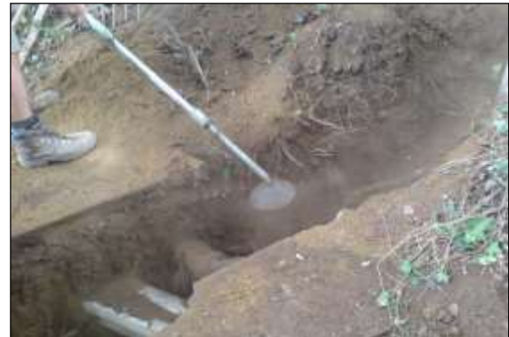
Photo 16: Air spades are very effective at exposing roots and services with minimal damage.
