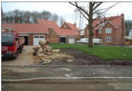
Photo 48: The RPA of this tree was not effectively protected during construction and excessive compaction of the soil meant it died soon after this turf covered up the damage.
