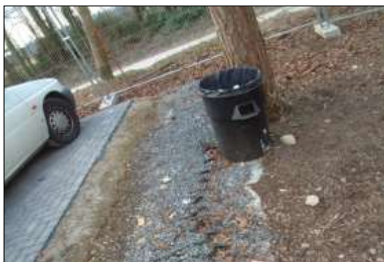
Photo 26: A conventional concrete haunching can be used to retain new surfacing as long as it is not dug into a trench - here is it placed on top of the CellWeb layer.
