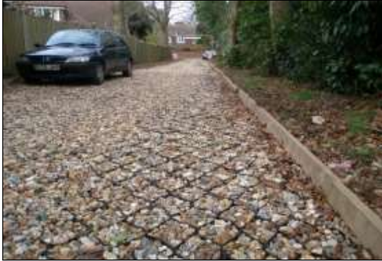
Photo 28: Wooden board pinned in place or held in position with backfilled topsoil can provide more informal and rustic surface edging.
