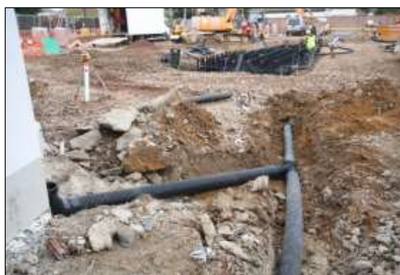
Photo 56: Drainage from adjacent buildings can be directed into Silva Cells, significantly buffering rainwater runoff from urbanised areas.
