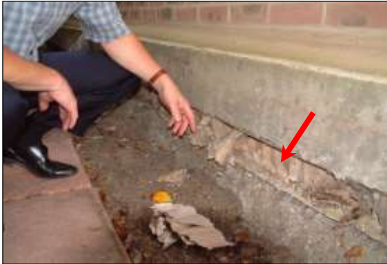
Photo 42: Where a slab is cast on site, a biodegradable void-former (red arrow) temporarily supports the weight of the liquid concrete until it sets. The void-former can then be wetted and washed away to leave a void or left to degrade naturally, both of which allow movement of air beneath the slab.
