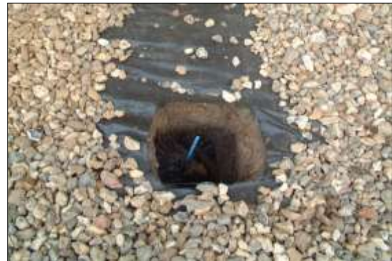
Photo 39: Ground protection must be used to spread the load of the piling rig once excavation has confirmed that no substantial roots are in the preferred pile location.
