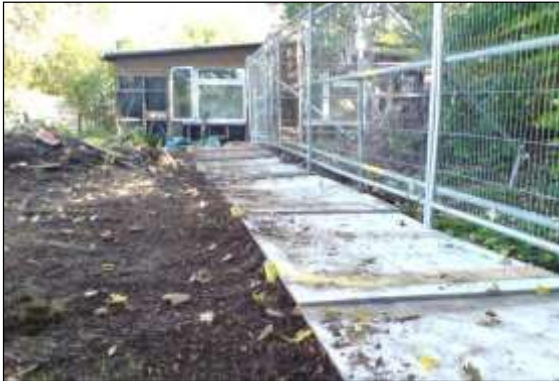
Photo 7: Heavy-duty plywood set onto a compressible woodchip layer and pinned into position is suitable to spread the loading from pedestrian access.
