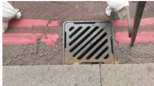
Figure 11 – Road gullies in front of the existing property
