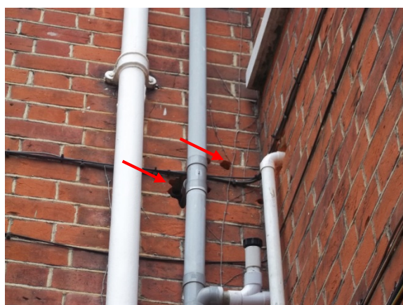
Plate 3.13: Damaged brickwork
