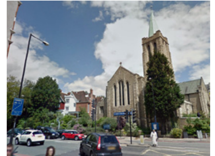
4. View towards the site from the junction of West End Lane
